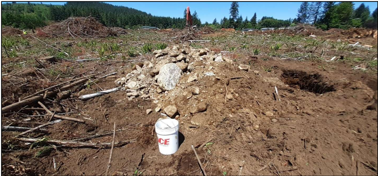
Typical Excavation Spoils Observed, TP-3
