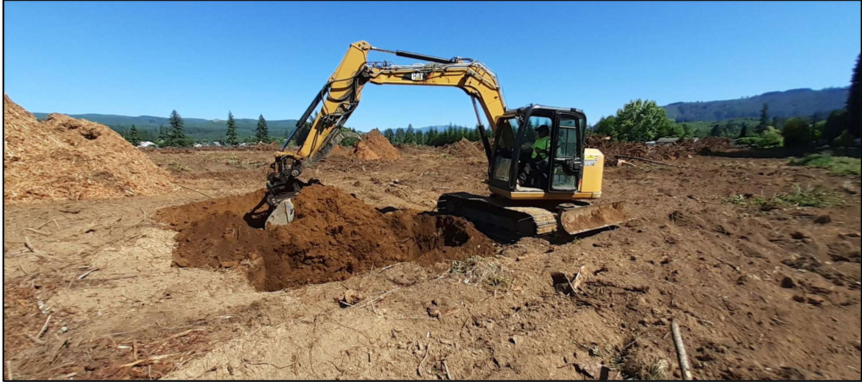
Conducting Test Pits, TP-6
