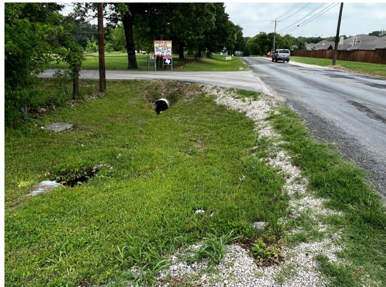
Lack of Sidewalks Along Stone Road
