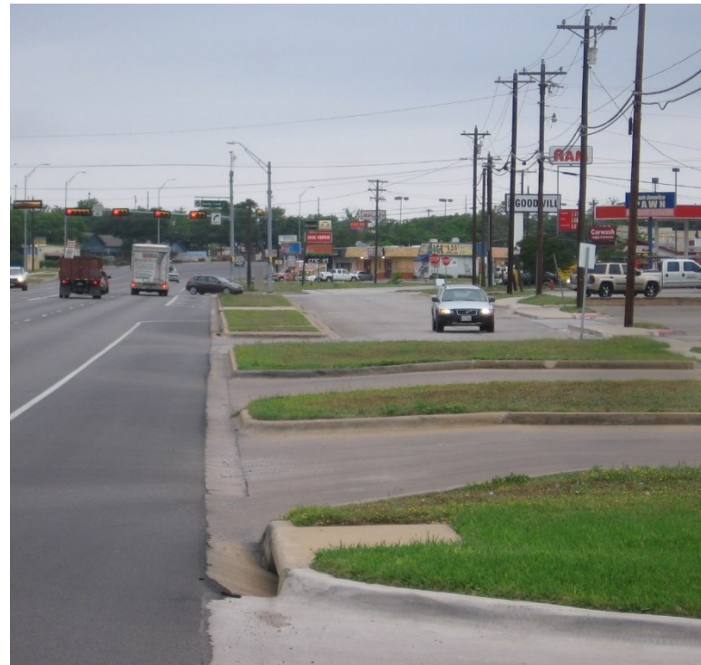
Example of Excessive Curb Cuts
