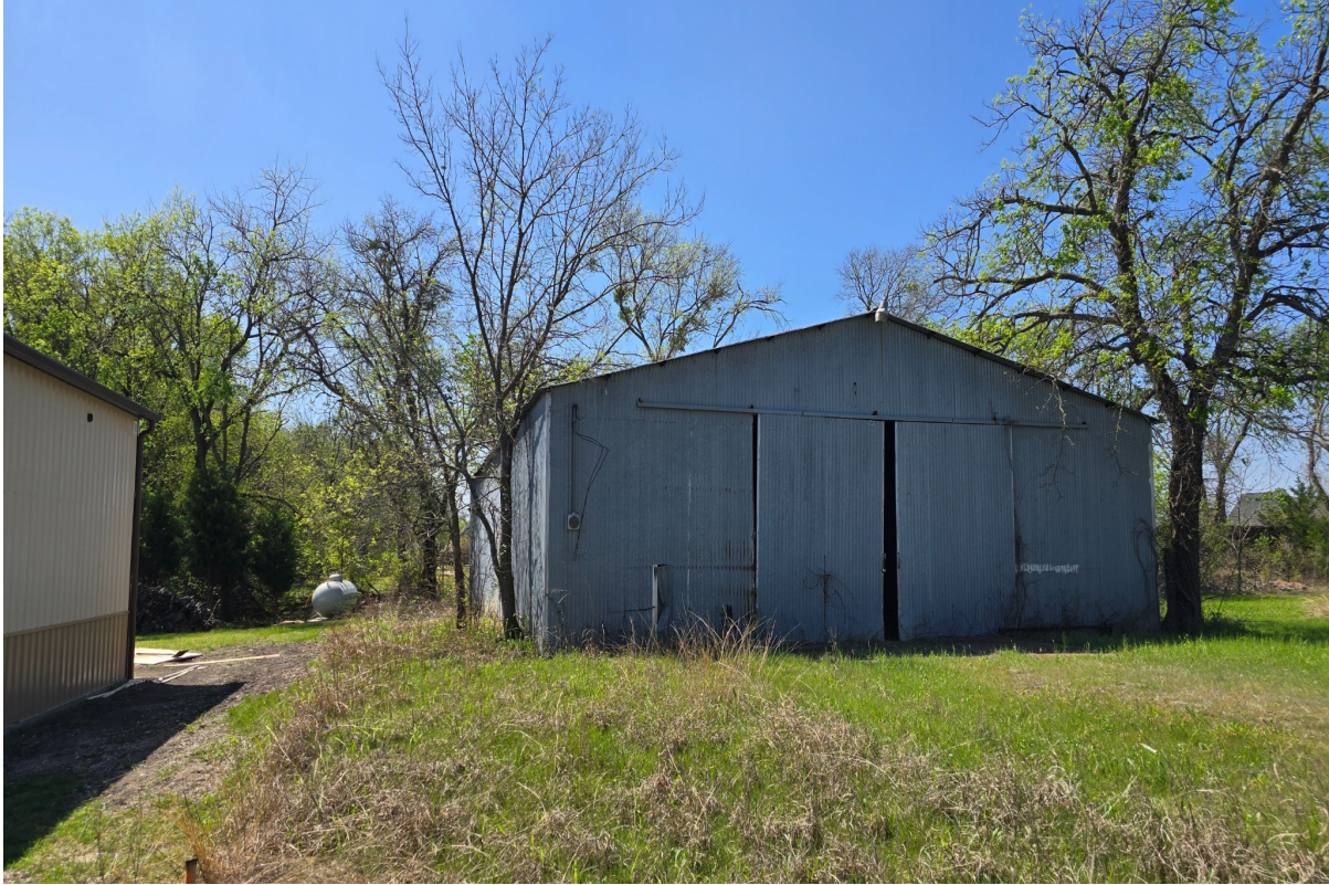
Exterior View – Overall Structure
