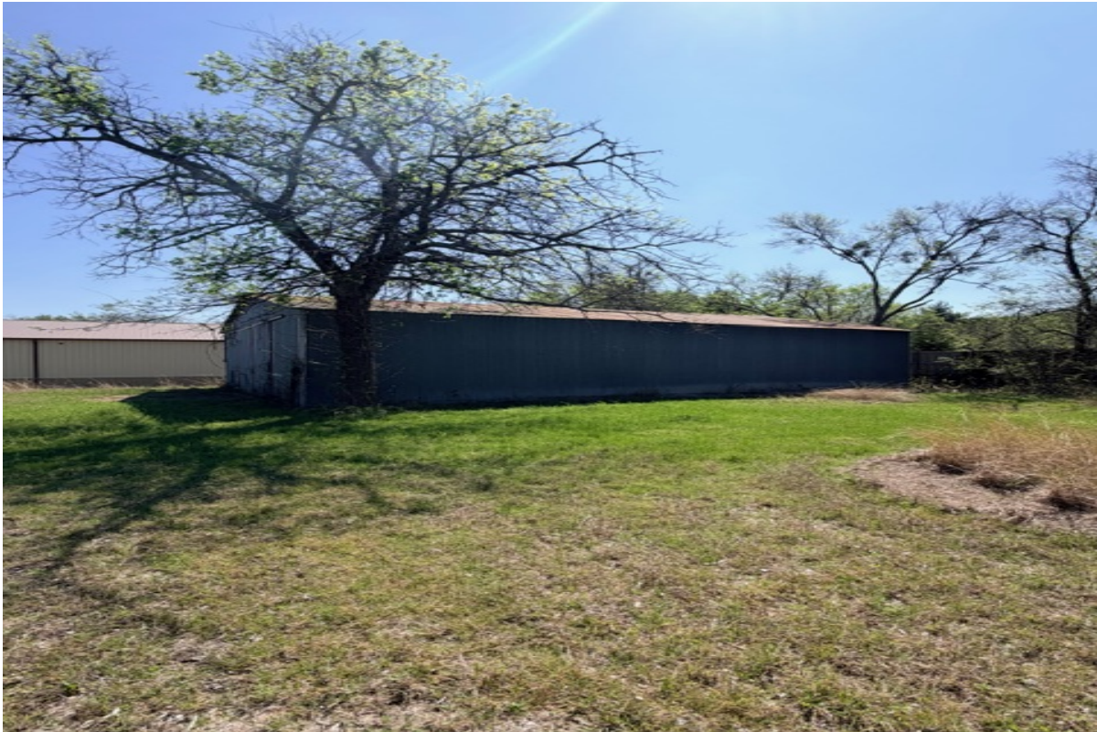
Exterior View – Side Elevation
