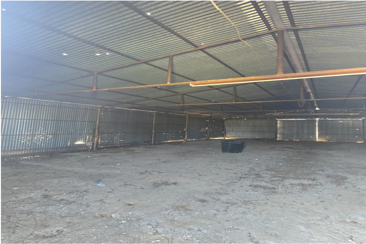
Interior View – Roof and Framing
