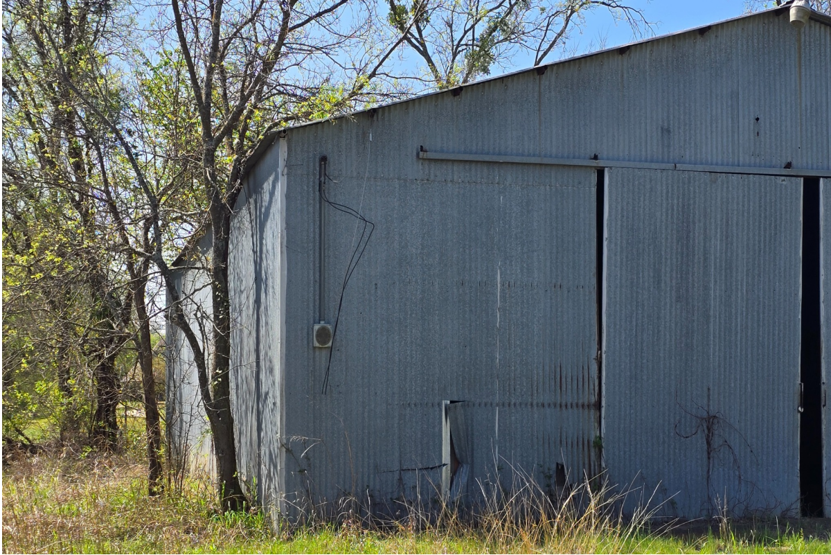
Exterior View – Rear/Side Condition
