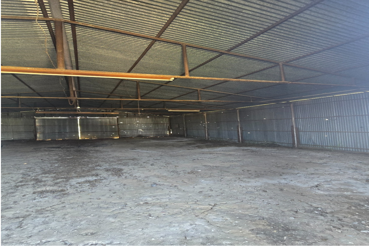
Interior View – Structure Condition
