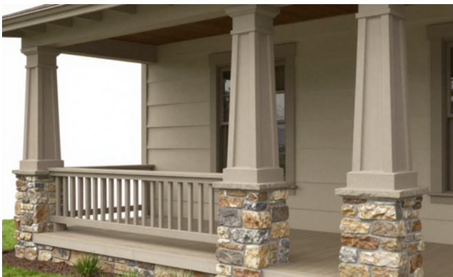
Tapered Columns on Stone Piers
