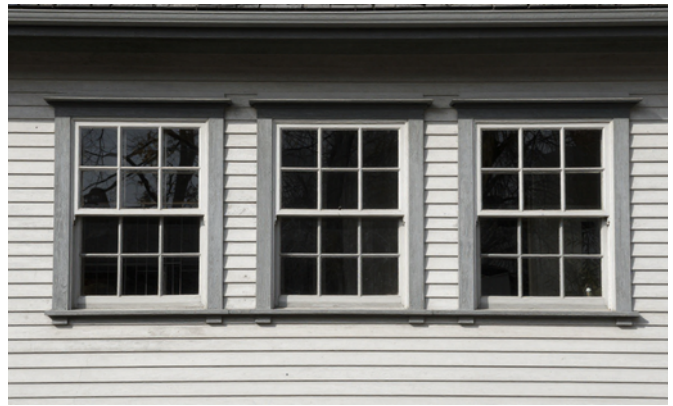
Banded Casement Windows
