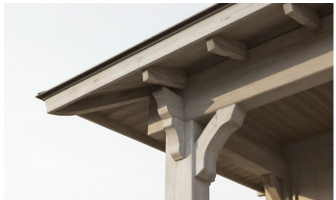
Exposed Rafters / Knee Braces
