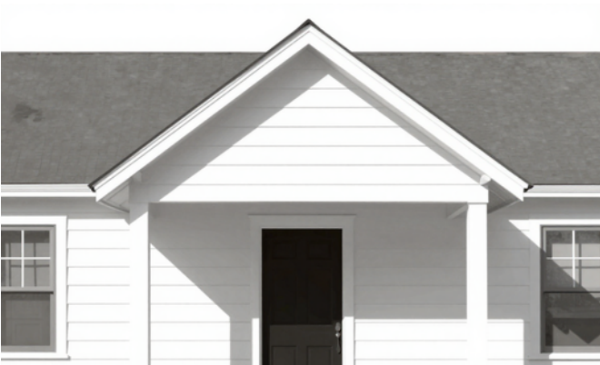
Front Cross-Gable Entry & Small Porch
