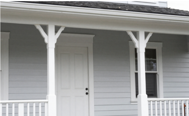
Front Porch with Tapered Supports
