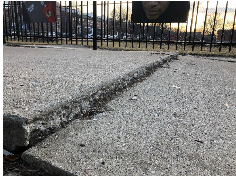
Sidewalk Requiring Repair
