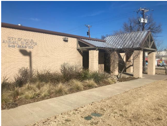
Front view of existing shelter
