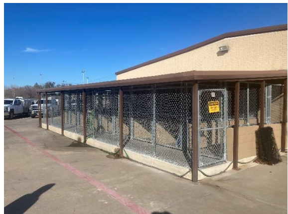
Side of Existing Shelter showing Existing Outdoor Dog Kennels
