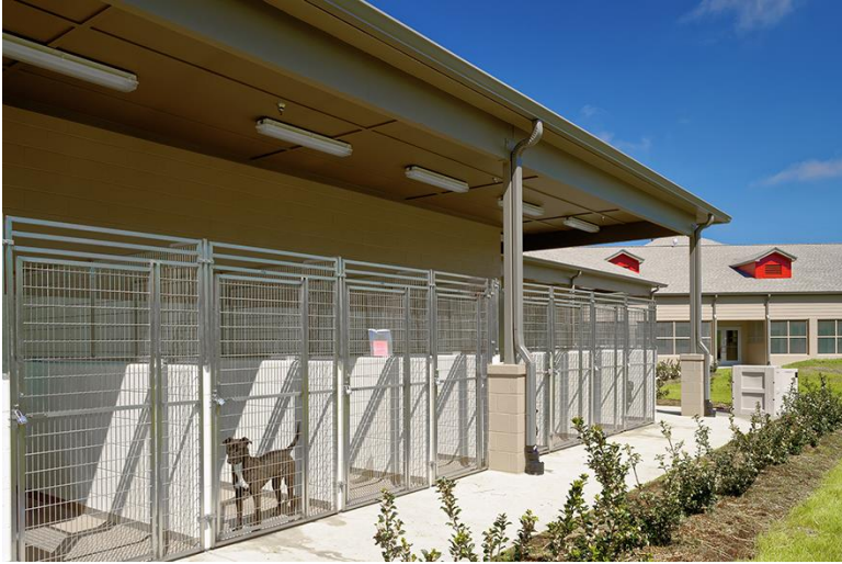
Photo of outdoor portion of indoor/outdoor kennels Note: Wylie intends to have the overhang extend out to cover the outdoor walkway in front of the outdoor Kennels.
