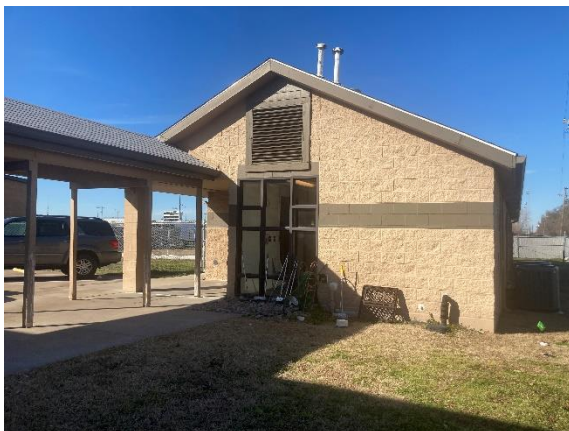
Front of Dog Kennel Building
