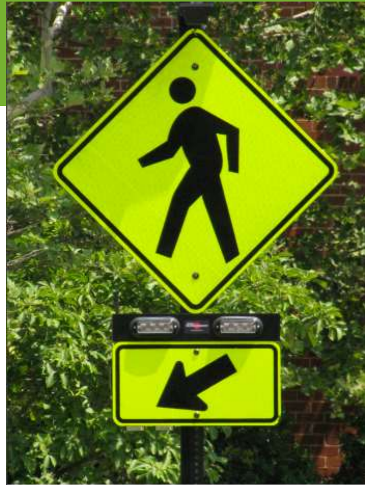
A Rectangular Rapid-Flashing Beacon (RRFB). Source: Carol Kachadoorian (2012) pedbikesafe.org
