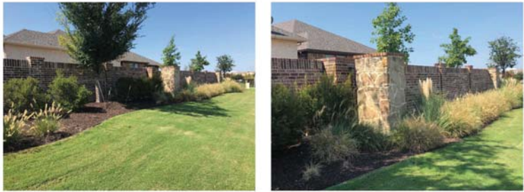
6'-0" HT. MASONRY SCREENING WALL WITH COLUMNS EXAMPLE PHOTOS NOT TO SCALE
