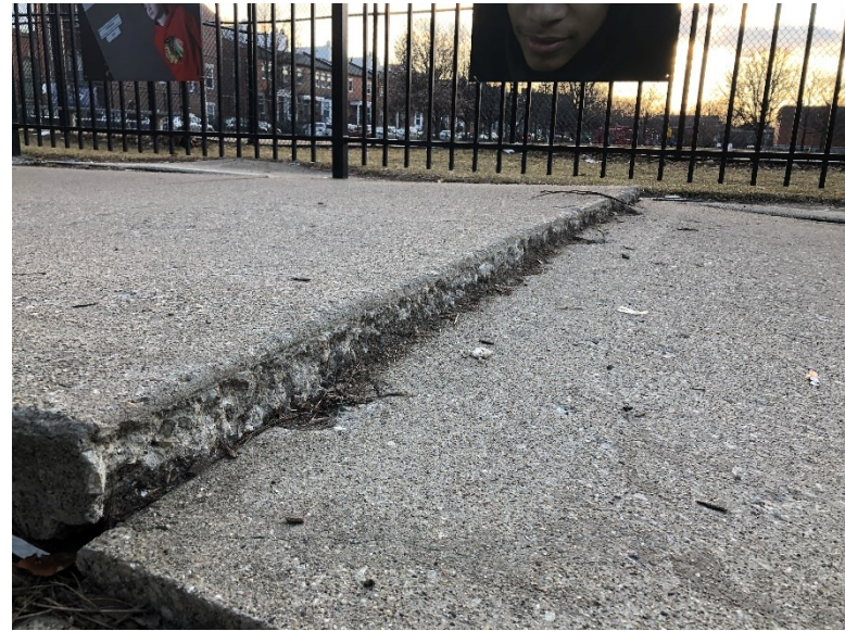
Sidewalk Requiring Repair
