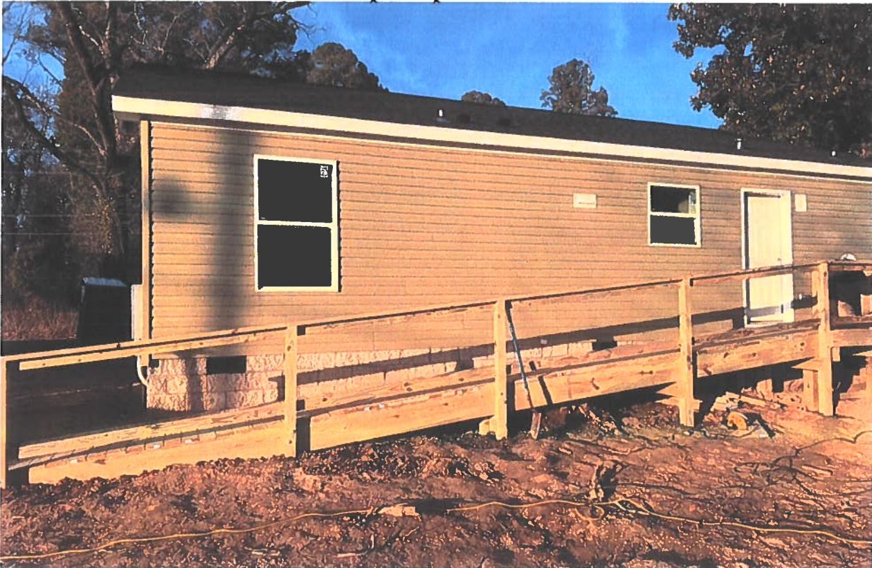
150 Meadowbrook Road – Access Ramp Completed:
