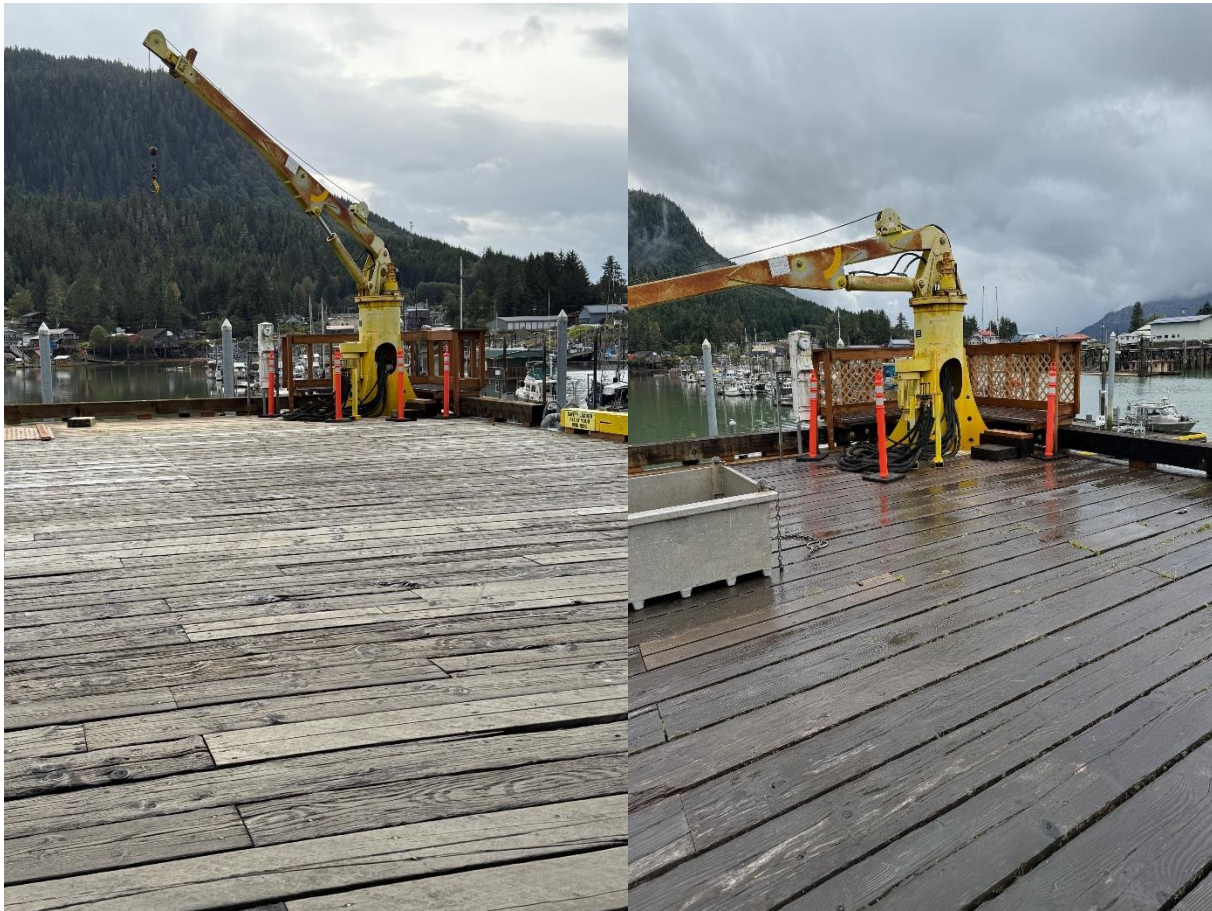
Reliance South crane bullrail and safety rail replacement:
