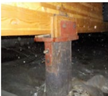
Typical creosote treated timber piling beneath 1988 addition, below emergency room. In good condition.
