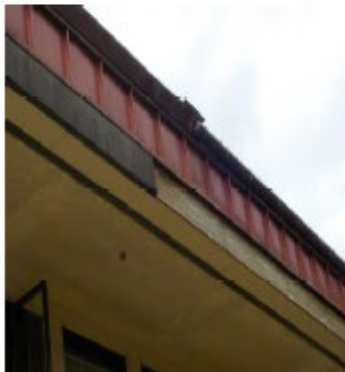
Deficiency Item S05. Missing EIFS fascia.
