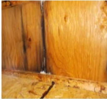
Deficiency Item S01. Minor roof leak creating moist condition for mildew growth (white).
