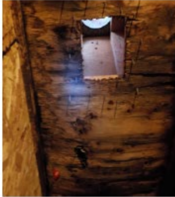
Deficiency Item S01. Decayed plywood roof sheathing typical at (2) roof ventilation turrets. Nontypical condition of framing.
