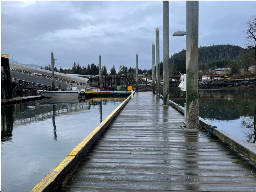
Photo 1. Overview of gangway/breakwater float
