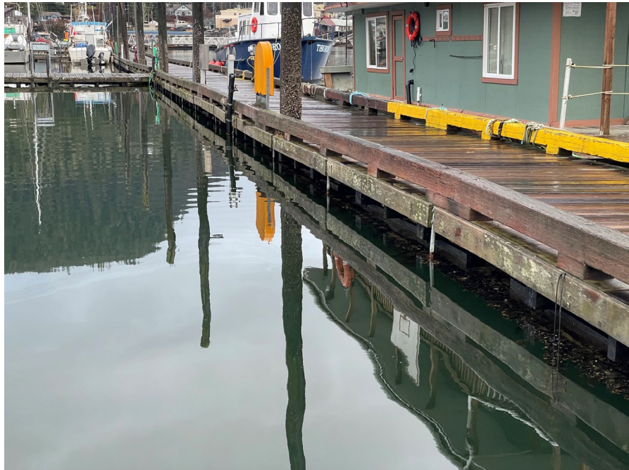
Photo 8. Overview of headwalk float
