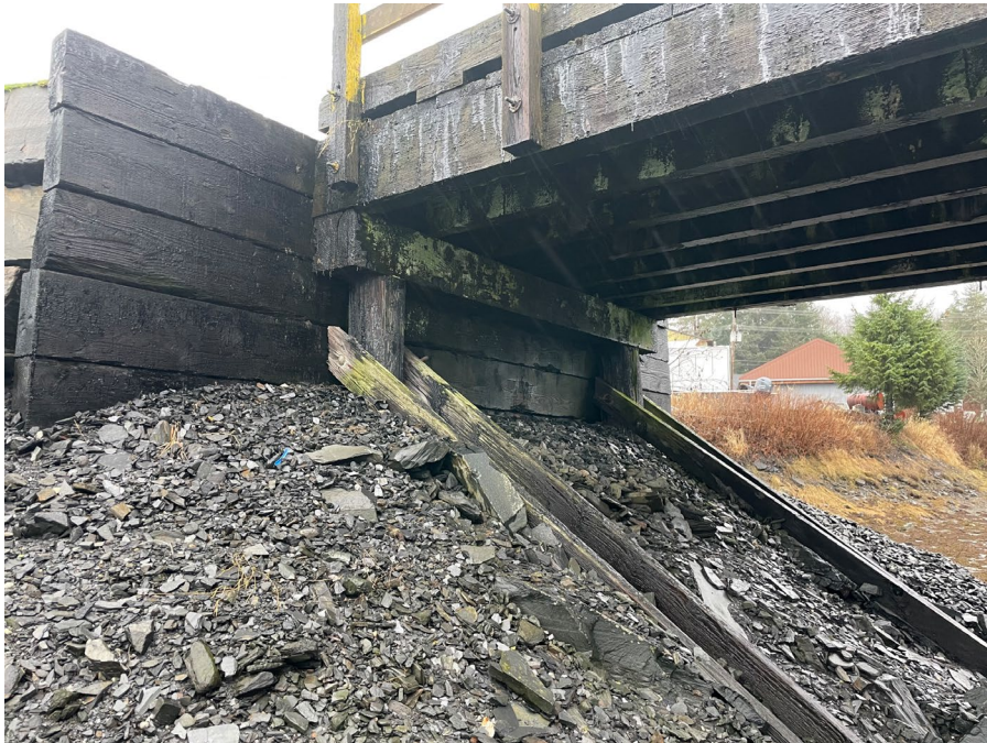
Photo 6. Timber backwall, stringers, pile cap
