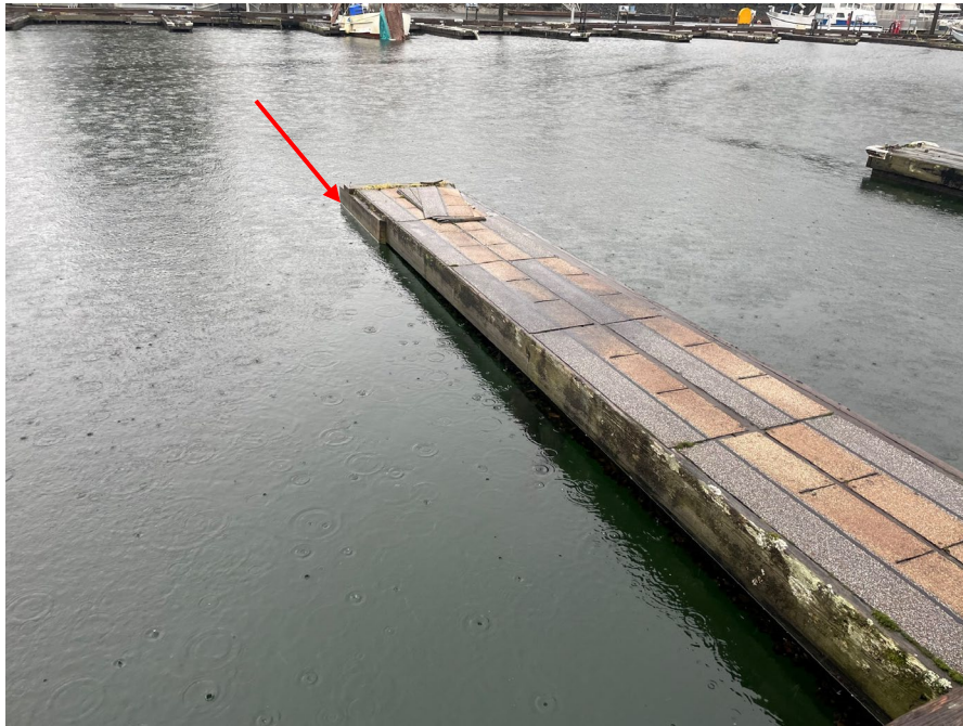
Photo 16. Loss of finger flotation at float end
