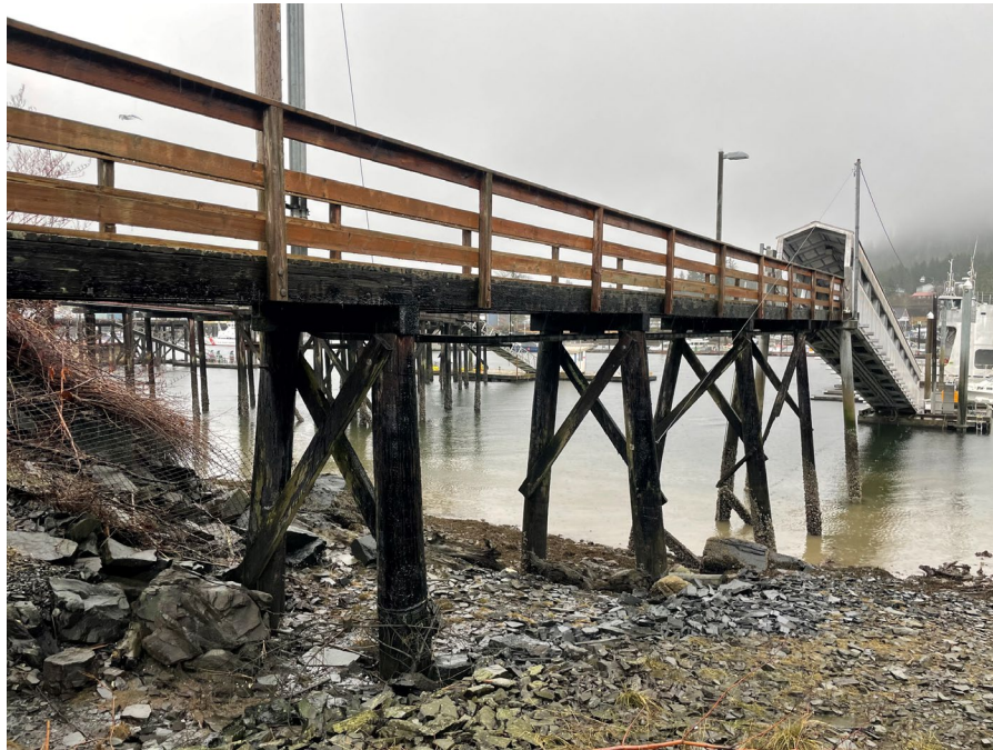
Photo 4. Profile of approach dock and gangway
