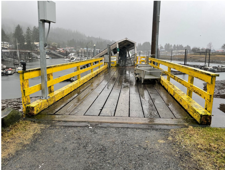
Photo 4. Topside of approach dock
