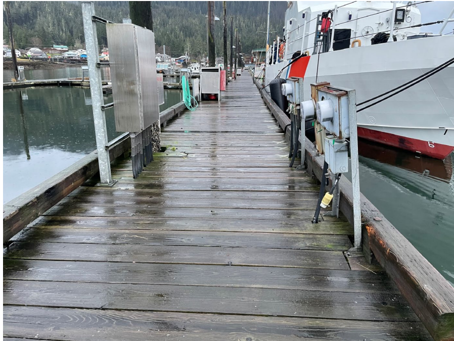
Photo 5. Overview of headwalk float
