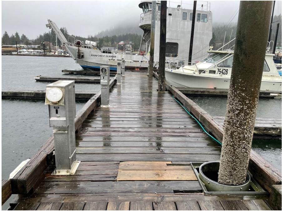
Photo 7. Overview of main float
