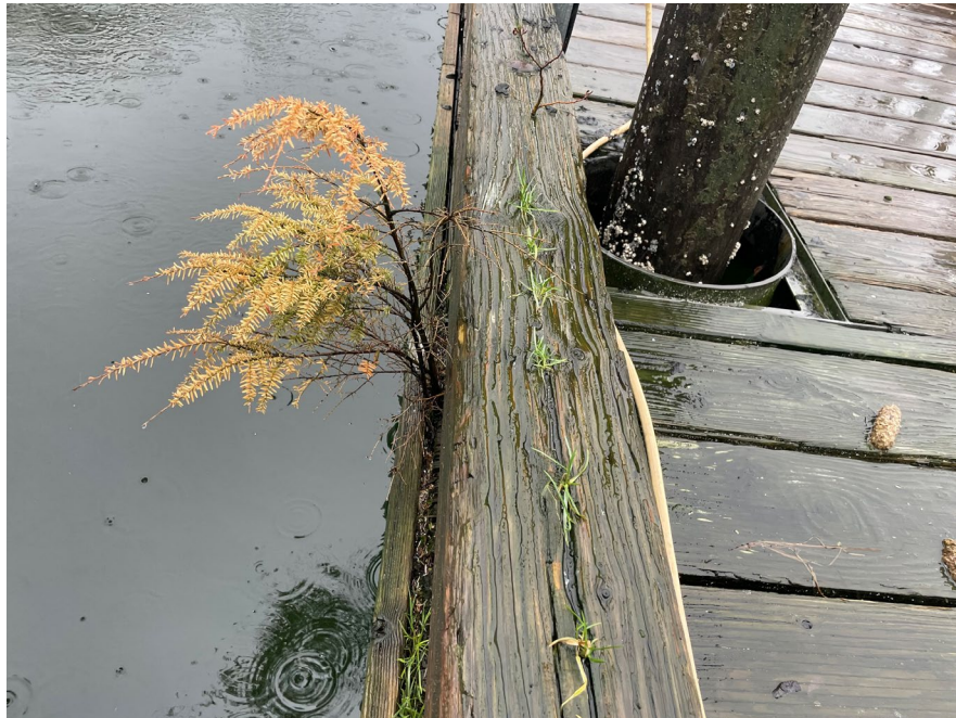
Photo 14. Typical moss/organics/plant growth on float timbers
