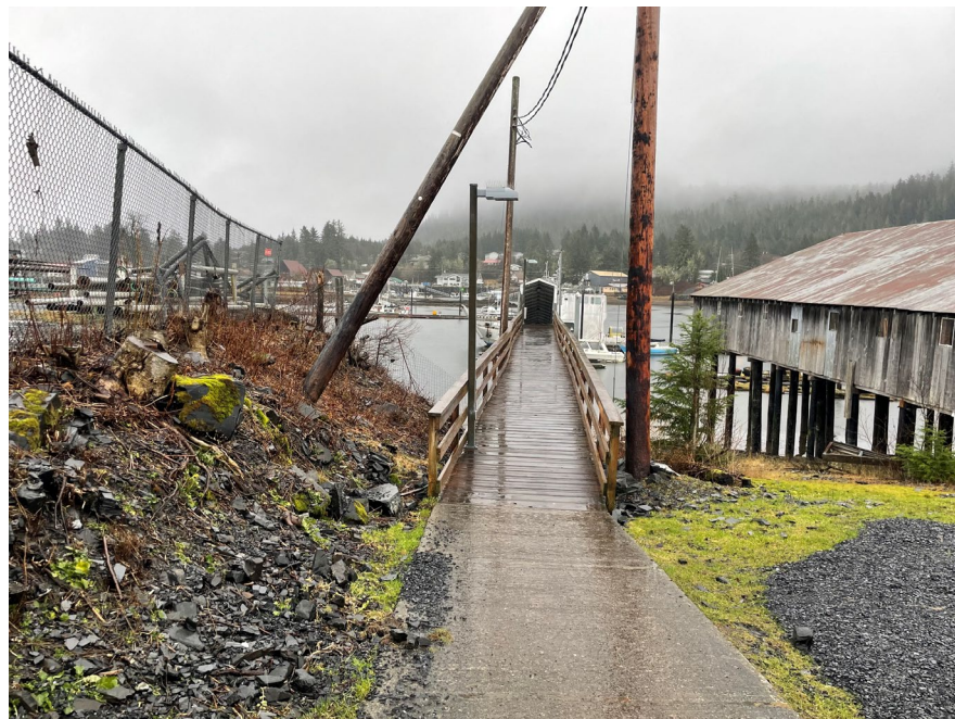
Photo 2. Overview of approach dock
