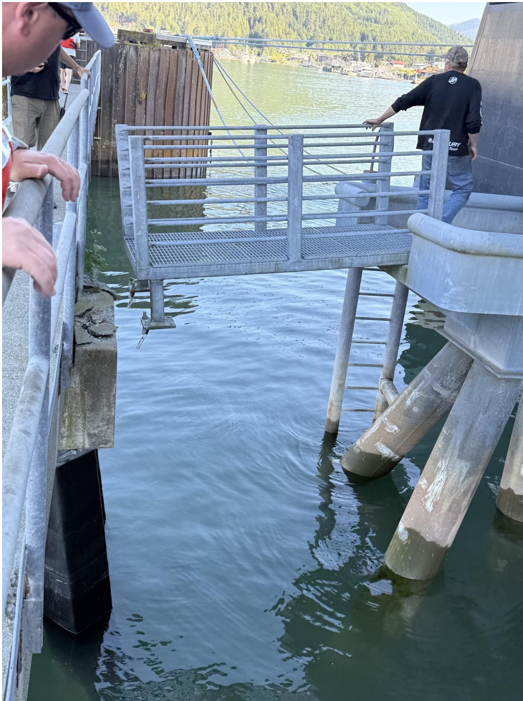
Photo 2. Closer view of the damaged area, including displaced/leaning dolphin piles and the adjacent access platform.
