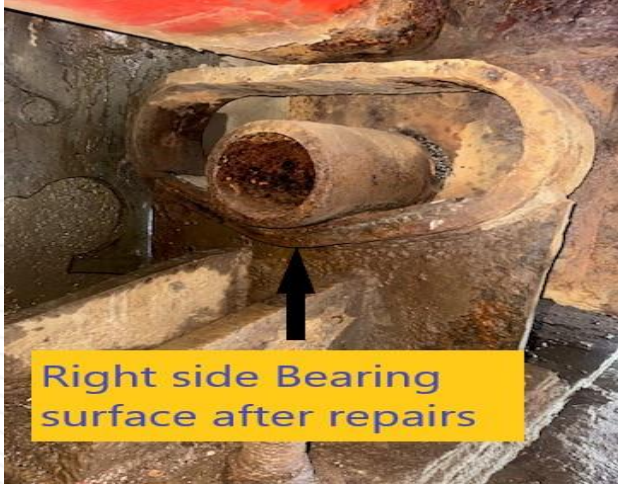
Barge Ramp Transition Repairs
