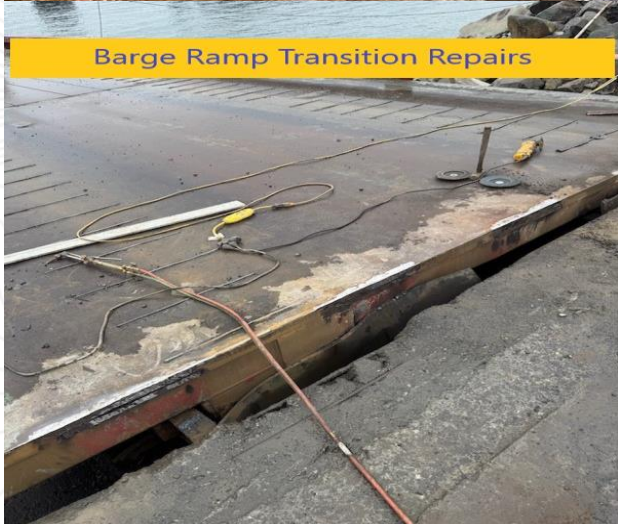
Right side Bearing surface after repairs
