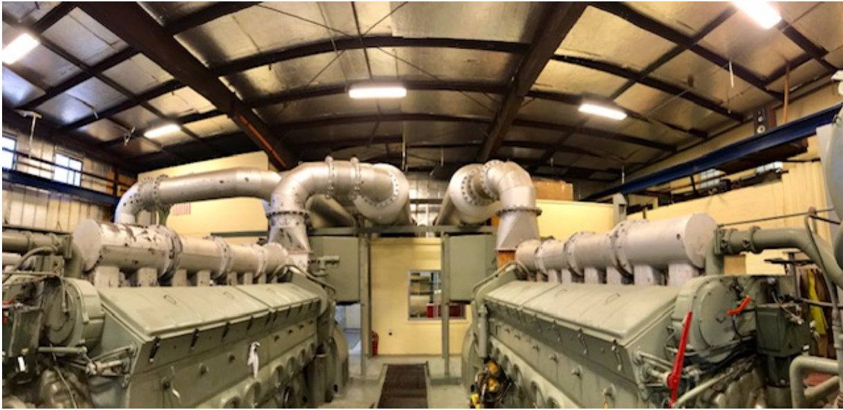
Three Existing Diesel Power Generators' Interior Exhaust Manifold View:
