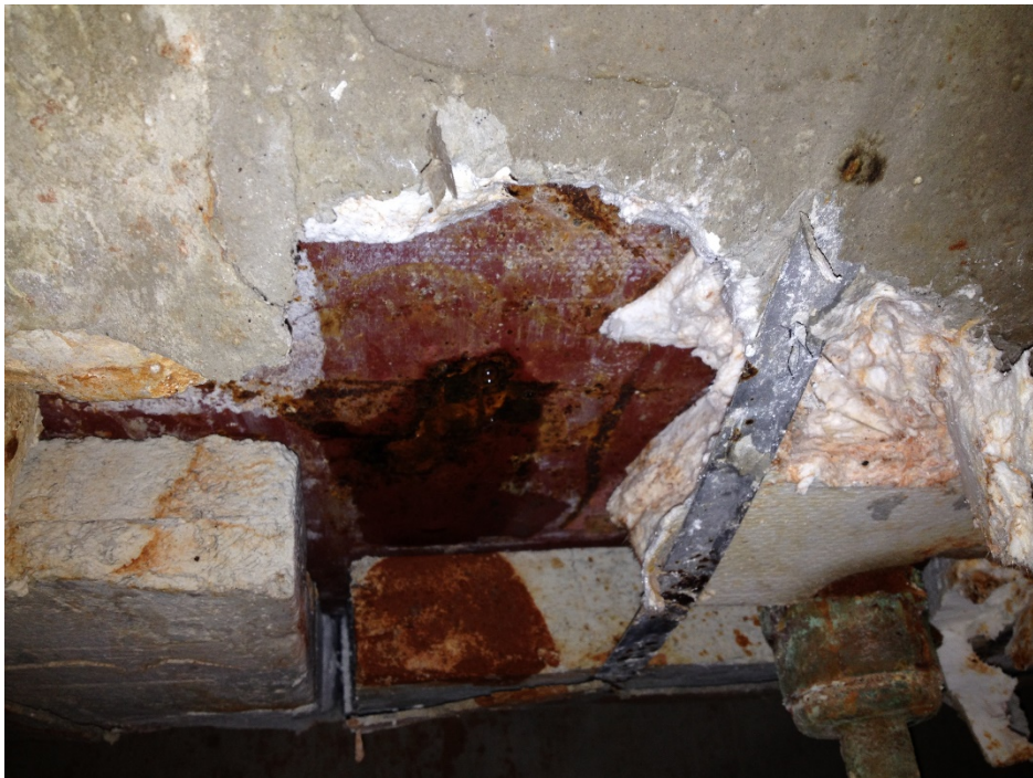
Sidewall Hole in Hot Water Tank:
