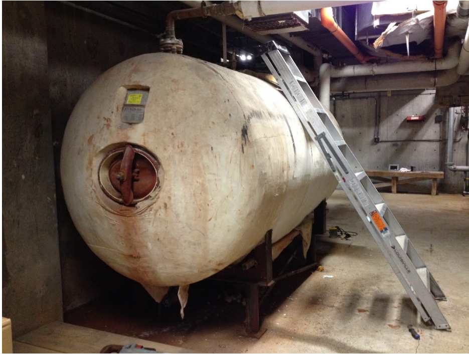
Existing 1200 Gallon Domestic Hot water Heater:
