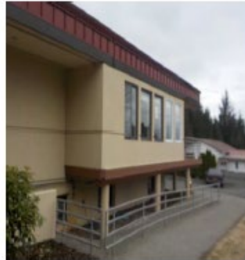
Deficiency Item S16. Addition bump out to activities room. Water runs down beneath the wall sole plate and runs across the floor. Foundation piers have settled.
