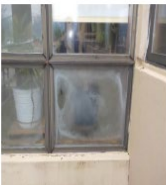
Deficiency Items S06, S07 and S08. Example damaged EIFS (freeze-thaw), fogged window, caulking sealant failure, siding in need of exterior paint
