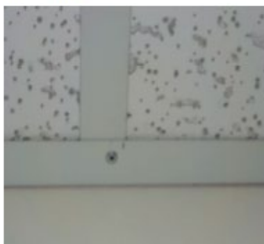
Deficiency Item S12. Rooms over 144 sf, metal grid runners are fastened to angle on all four sides of ceiling. Only one side shown in photo.
