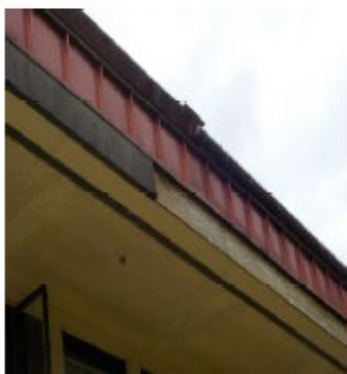
Deficiency Item S05. Missing EIFS fascia.
