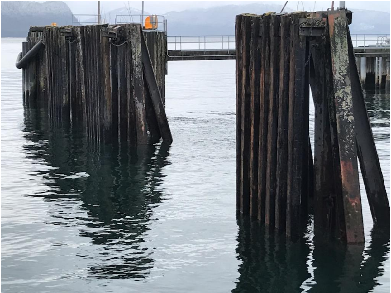
H Pile Dolphins and Fender Piles
