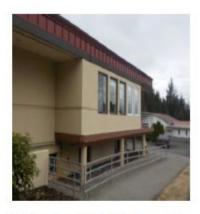
Deficiency Item \$16. Addition bump out to activities room. Water runs down beneath the wall sole plate and runs across the floor. Foundation piers have settled.
