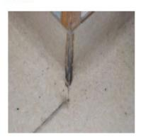
Deficiency Item S11. Example vinyl Flooring seam failure.
