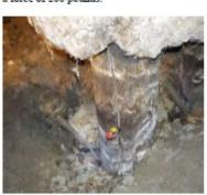
Deficiency Item \$17. Decayed creosote treated timber piling. Nontypical condition, not representative of average piling condition. Most pilings were found to be in good condition.
