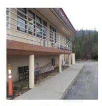
Deficiency Item \$15. Note dip in deck rim board. Guardrails non-code compliant. Space between horizontal rails exceeds 4". Connection to deck not capable or resisting a force of 200 pounds.
