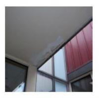
Deficiency Item S04. Example water damaged roof soffit sheathing.
