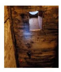
Deficiency Item S01. Decayed plywood roof sheathing typical at (2) roof ventilation turrets. Nontypical condition of framing.
