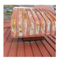
Deficiency Item S03. Air handler hood with corrosion.
