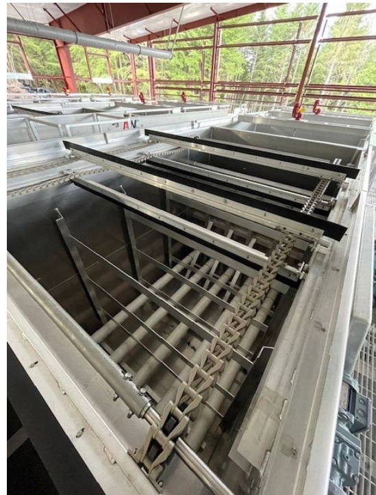
WTP - View into one of the DAF basins:
