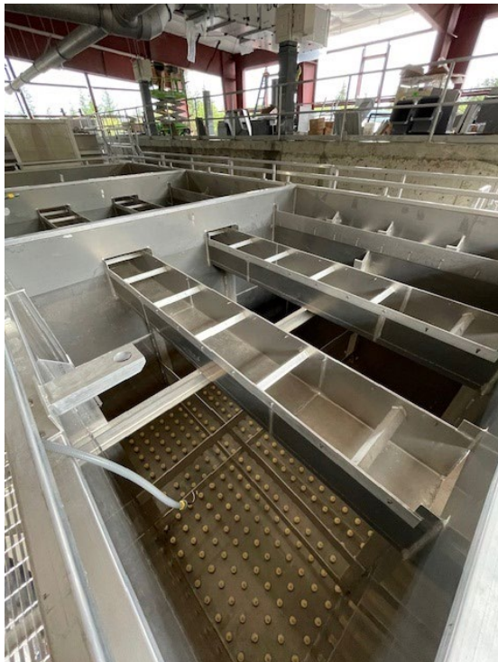
WTP - View into one of the Filter basins:
