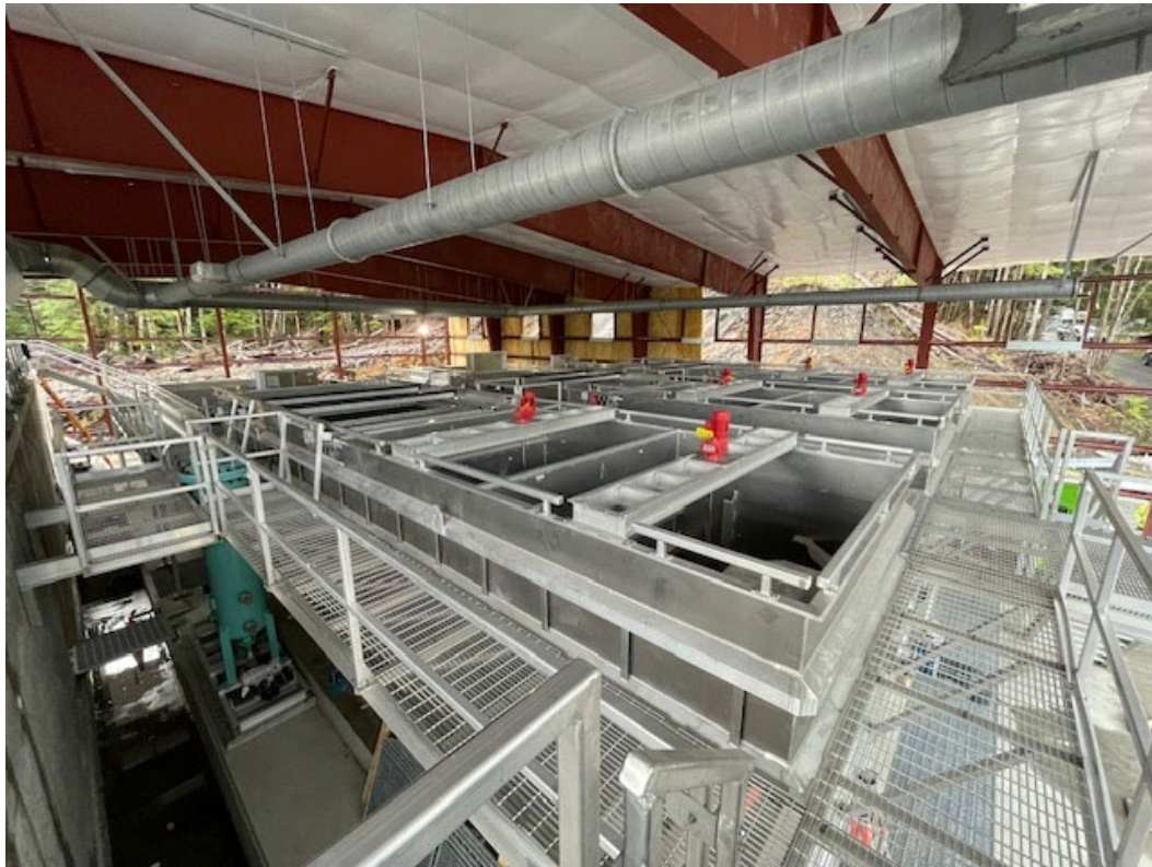
WTP - View into one of the Filter basins:
