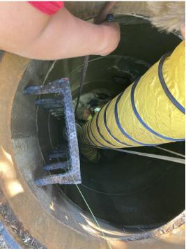
Forced mains keep the sewer lines fairly clear due to the high flows that go through them. Gravity fed mains are more likely to clog over time. We especially run into issues if there is a sag in the main. In these instances it can be difficult to clear the sag and push those materials through to where they can gravity feed or be removed.
