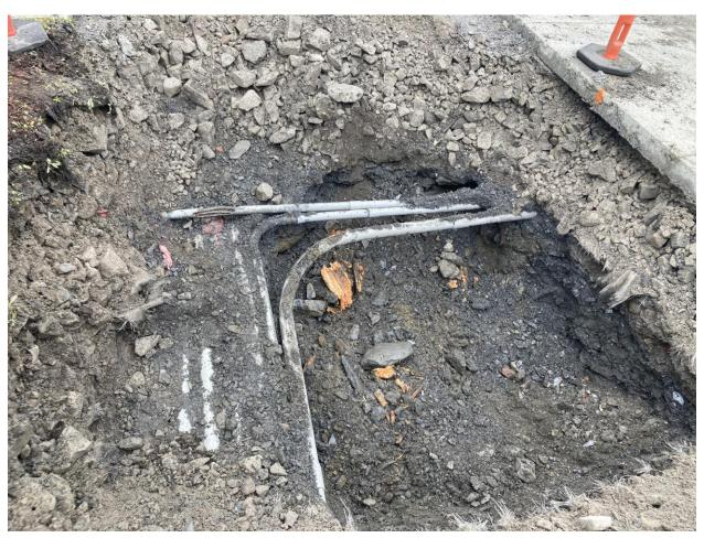
Another value of having a vac truck when working on water mains is the fact that water mains can stay in positive pressure while they are worked on.
