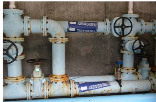
22) Filtered water piping in the slow sand filter building.
