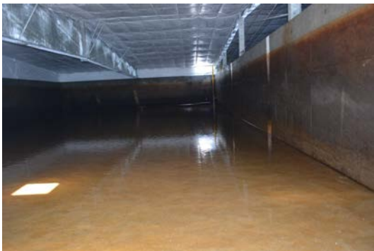
19) This is the interior of slow sand filter #4, which was drained and opened for inspection on April 15.
