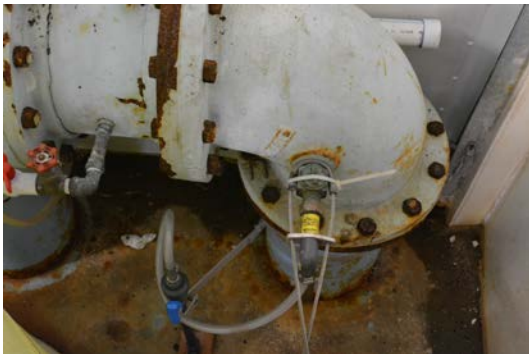
7) The sodium hypochlorite injection point is located just behind the Chlorotec generator. This line flows to the storage tanks.
