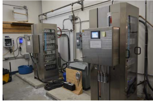
9) Both ozone generators were replaced in 2017. These units were never programed for proportional dosage control by the flow meter.
