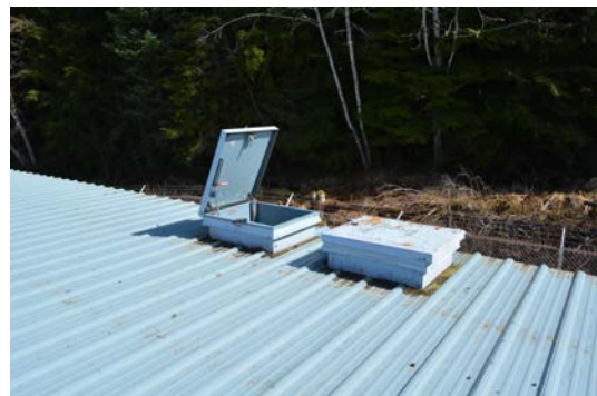
16) Access hatches for each of the slow sand filters are located on the roof of the filter building.
