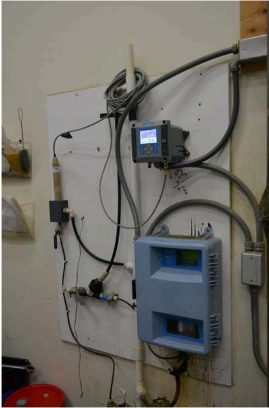
24) The finished water online pH and chlorine residual analyzers are located inside the ozone generator room in the operations building.
