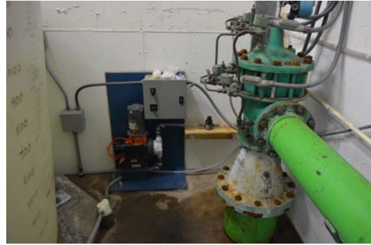
4) Caustic soda dosing pump.
