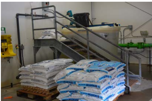
3) Caustic soda solution tank for pH adjustment of the raw water entering the operations building.
