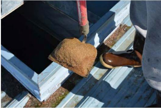
18) This was the sand filter skimming sample from filter #4.
