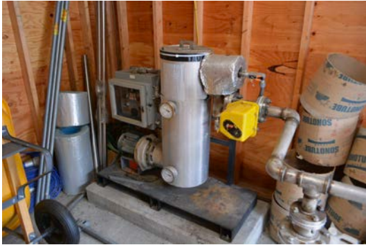
12) Ozone off gas is converted back into oxygen in two ozone destructors in the ozone diffuser building.
