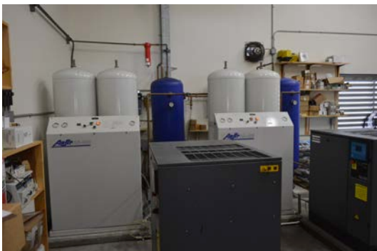
8) The ozone system air compressors and associated equipment are also located in the operations building.
