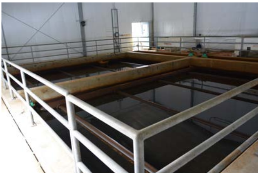
14) View of the two roughing filters from inside the roughing filter building. These are upflow filters with a top layer that had to be rebedded with coarser river gravel to provide an adequate flow rate.
