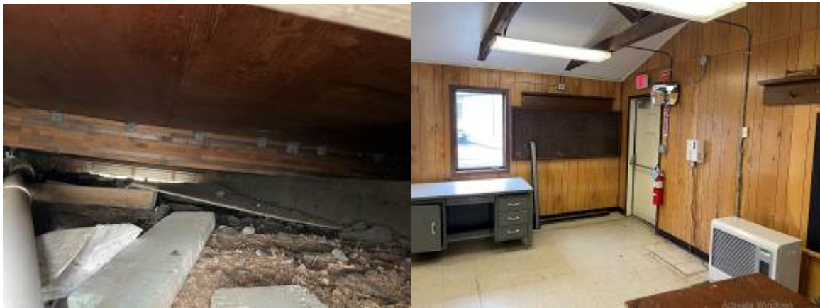
Above left is the underside of the building and as can be seen the subject is sitting on wood grade beams. Above right is a view of the interior looking at the NE corner. The oil fired Toyo heater is viewers right.
