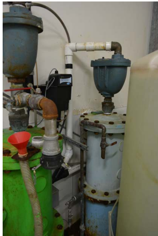
5) An on-line Hach 1720 filtered water Turbidimeter (center) is mounted next to the treated water (blue) riser pipe on the right.
