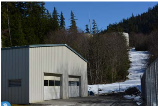
25) The finished water storage tanks are located on a hill above the WTP. These have a combined capacity of 0.85 million gallons. The Wrangell distribution system maintains flow and pressure by gravity from these tanks.
