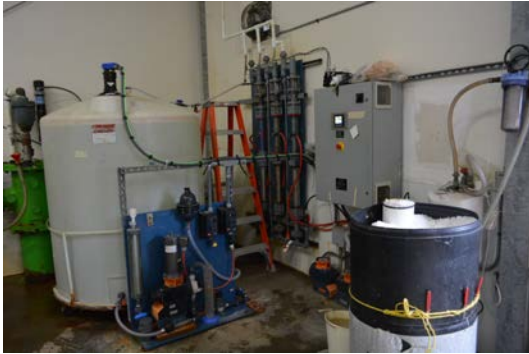
6) The Chlorotec onsite sodium hypochlorite generator (center on wall) and solution tank (left) are also located inside the operations building.
