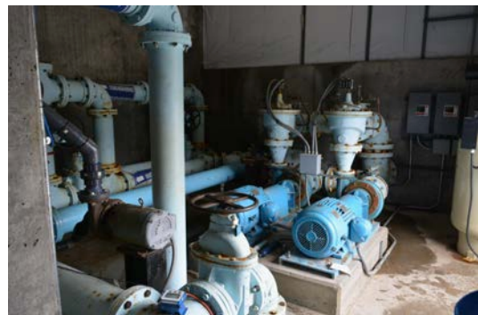
23 Filtered water pumps in the slow sand filter building. These are each rated at 900 gpm.
