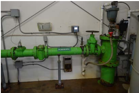
2) Raw water inlet in the operations building. The tap on the vertical riser on the right was used for raw water samples in this project. This is the tap that was used for the DAF pilot test in 2016. The caustic soda injection point is to the left of the gate valve.
