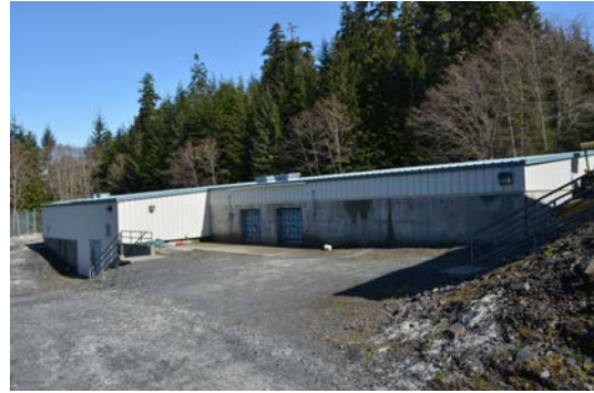
15) The slow sand filter building houses four filters, each with a surface area of 3,040 square feet.
