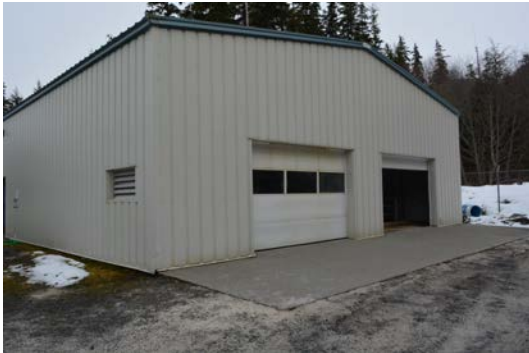
13) Roughing filter building. This building had to be ventilated before it could be entered to remove ozone released above the filters.
