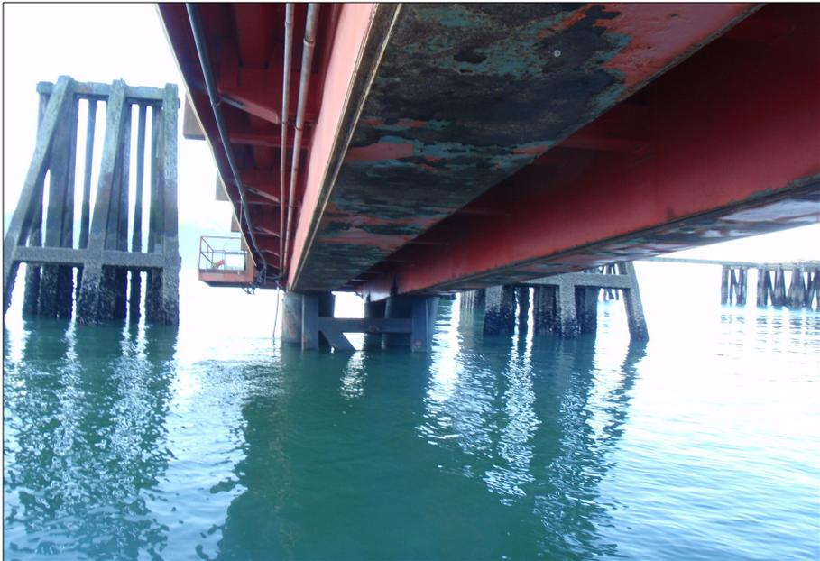
43 Ramp box-girder bottom flanges; coating failure, minor corrosion, typical.
