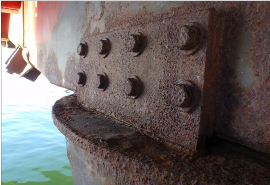
Coating failure/corrosion at ramp/support tank connection assemblies.
