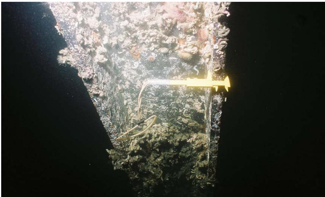
**PHOTO No. 13:** Breasting Dolphin C, Pile 3 Batter – Note the yellow caliper on the flange at this Level II cleaned site and the good condition of the epoxy coating in the submerged zone.
