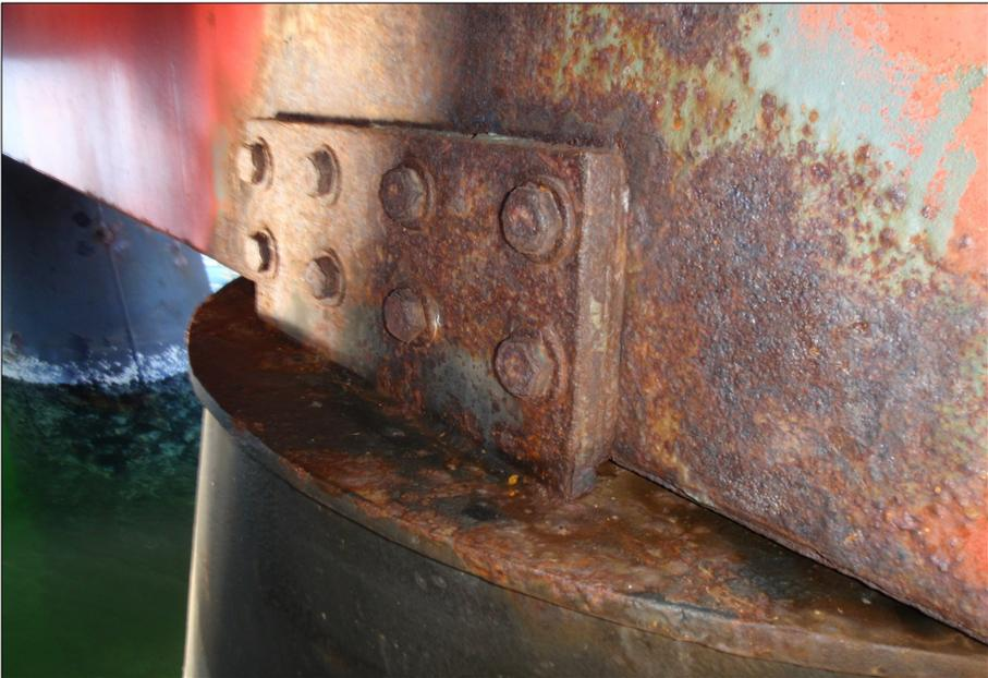
Coating failure/corrosion at ramp/support tank connection assemblies.
