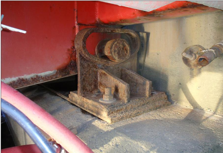
South bearing assembly; coating failure on all steel components.
