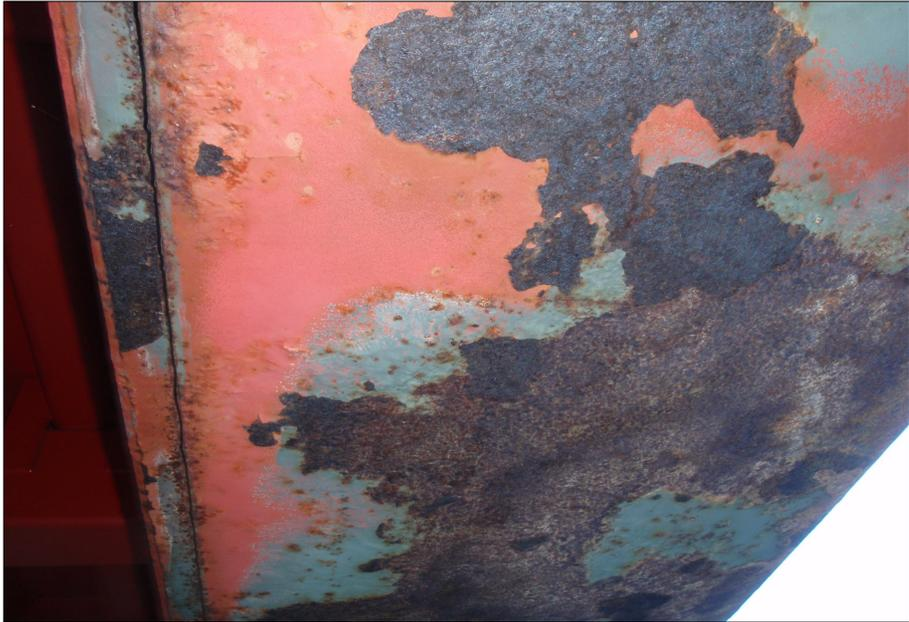
Typical coating failure/corrosion of girder bottom flange.
