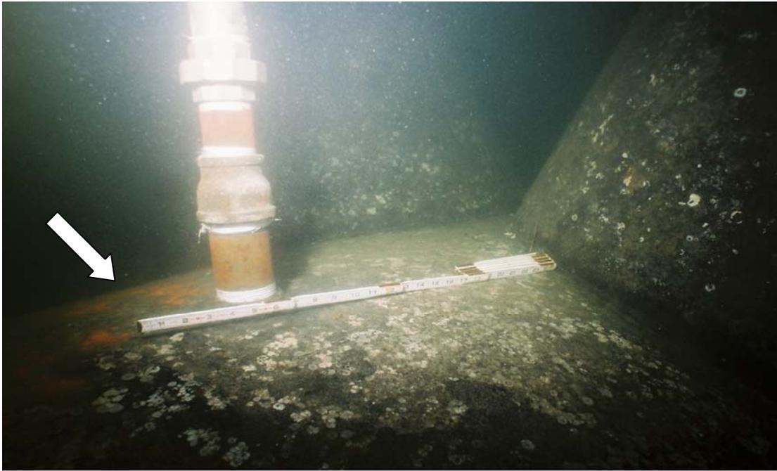
**PHOTO No. 7:** Floatation Tank, Air Inlet Port – Note the good condition of the air inlet port located at the south end at the crown of the 9 ft. dia. tank. Also note the good condition of the coating on the two pipe struts and the minor coating deterioration in the vicinity of the inlet.
