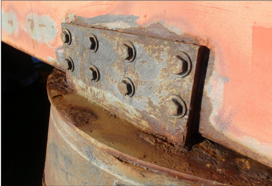
Coating failure/corrosion at ramp/support tank connection assemblies.
