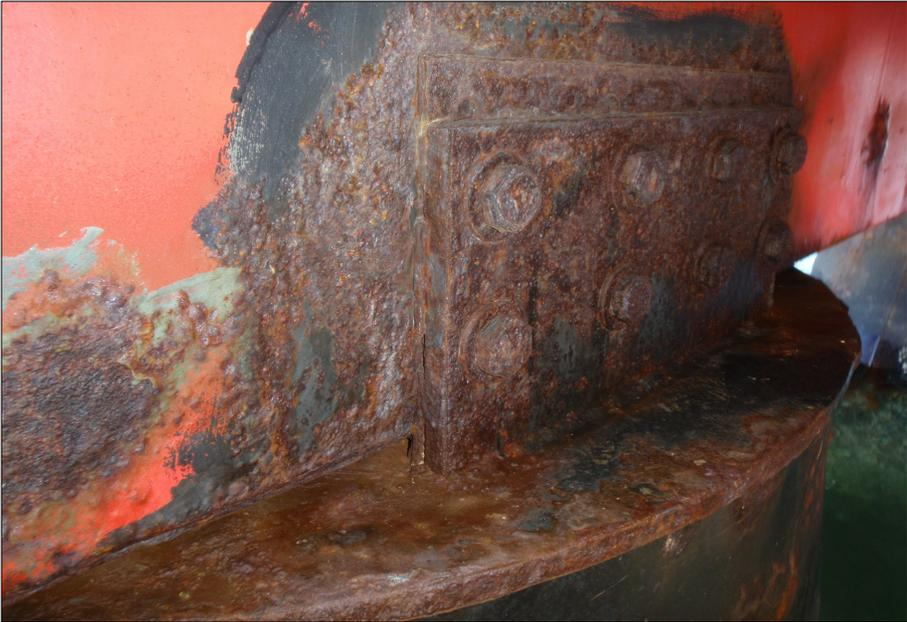
Coating failure/corrosion at ramp/support tank connection assemblies.
