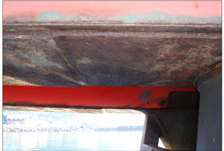
Typical minor corrosion of ramp girder bottom flange.
