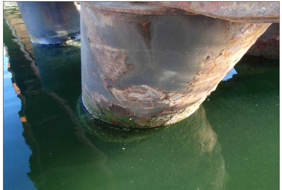
Typical coating failing/minor corrosion of ramp tank support strut.
