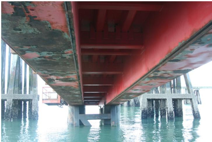
Figure 3 - coating failure along the barge ramp girder soffits
