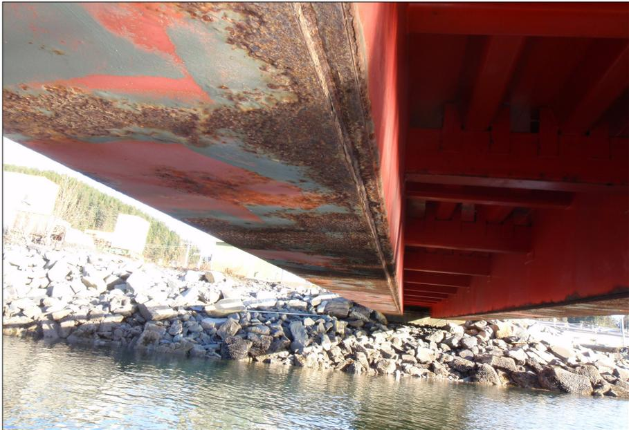
Ramp box-girder bottom flanges; coating failure, minor corrosion, typical.
