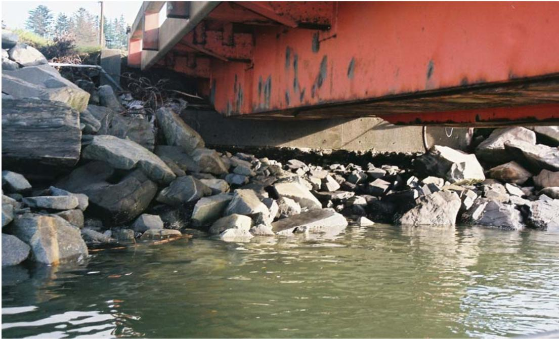
**PHOTO No. 3:** Transfer Span Bridge Seat – Note the undermining of the concrete bridge seat. Also note the localized failure of the painted coating on the transfer span members.
