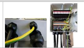
Feed cable into BTS – M40 cable gland is pre-mounted on the hybrid cable
