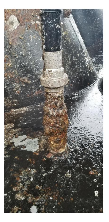
Corrosion to air inlet Floatation Tank
