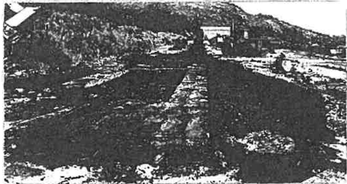
Figure 6: Looking south along the former green chain line area on 6/29/12. Excavations exposed 4'-wide foundations which later were discovered to be the former hydraulic-powered 'action pack'
