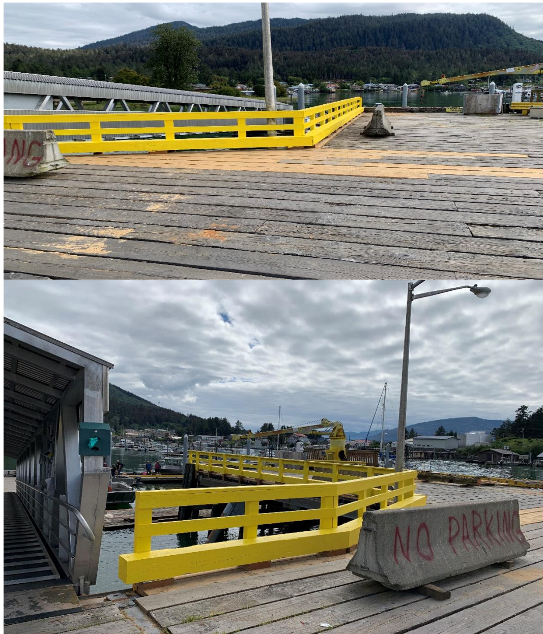
Figure 6 Finished Bull rail and Handrailing
