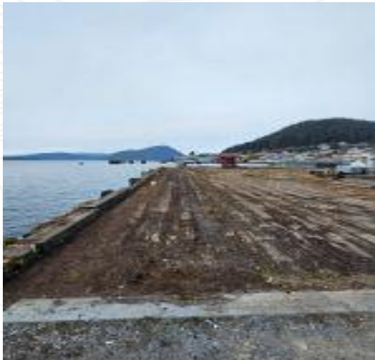
Figure 5 Mill dock Clean up
