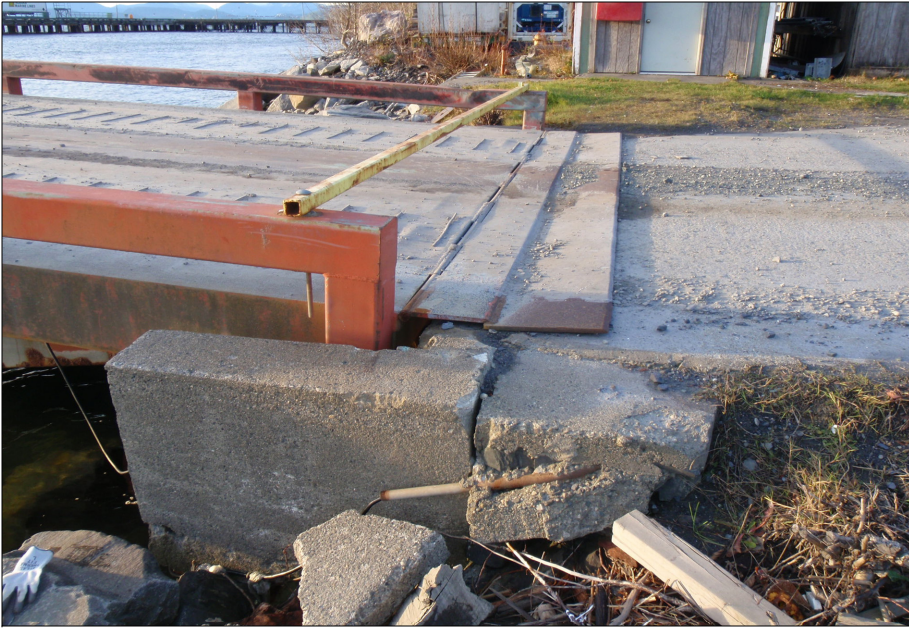
Transition plate at barge ramp abutment.
