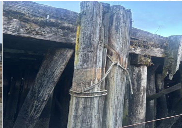
Figure 6 Mill dock Piling reattachment
