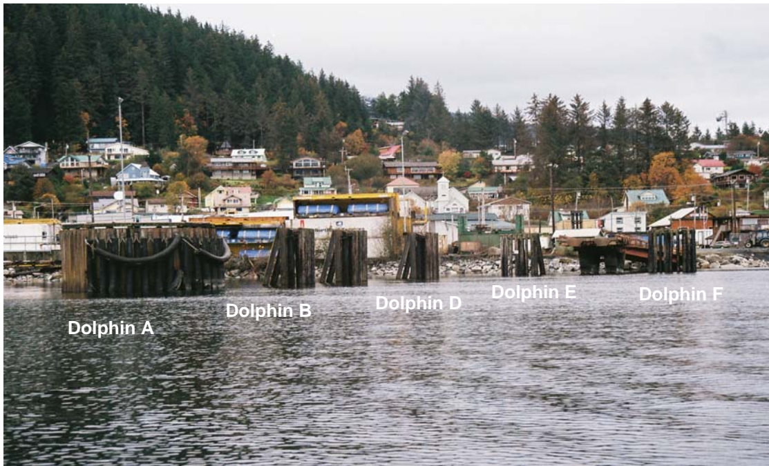
PHOTO No. 1: Wrangell Barge Facility Looking Northeast – Note the transfer span hinged off the shore. Also note the circular cofferdam, Dolphin A and the H-pile supported breasting Dolphins B – F.
