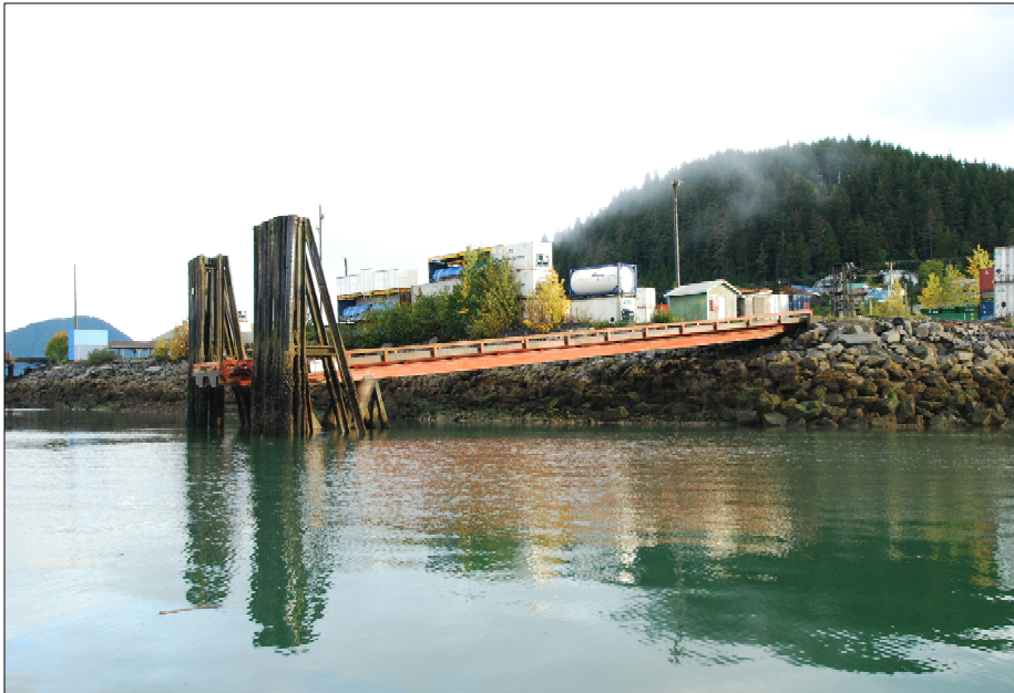
Overall barge ramp, looking north.
