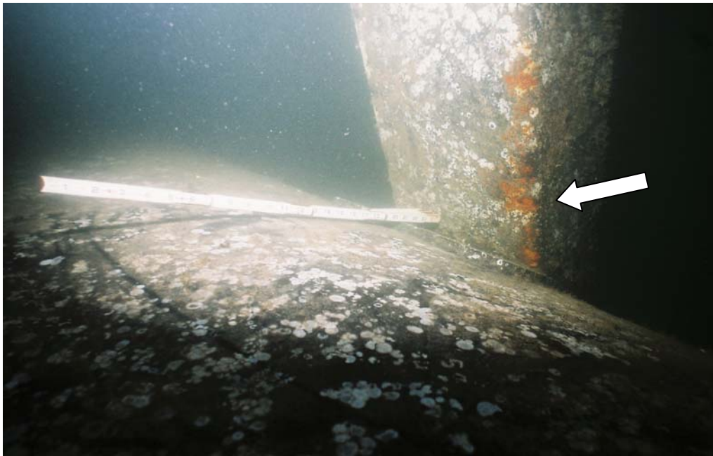
PHOTO No. 9: Seven Foot Diameter Floatation Tank – Note the good condition of the welded connection between the square tubular strut and the floatation tank. Also note the good condition of the epoxy coating on the top of the pontoon and the localized coating failure on the strut.
