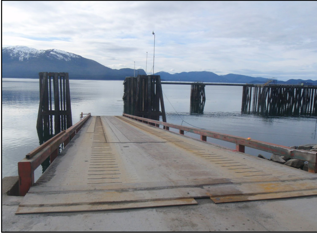
FIGURE 3. Barge ramp deck looking ramp from abutment.
