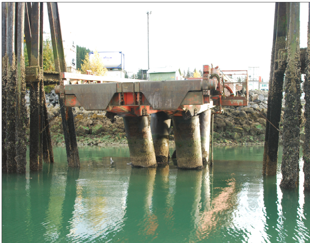
End of barge ramp, looking shoreward.
