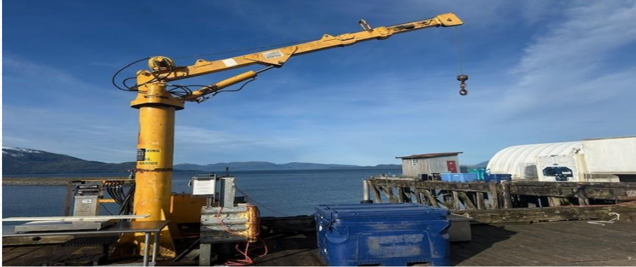
Figure 4 Mill Dock Crane
