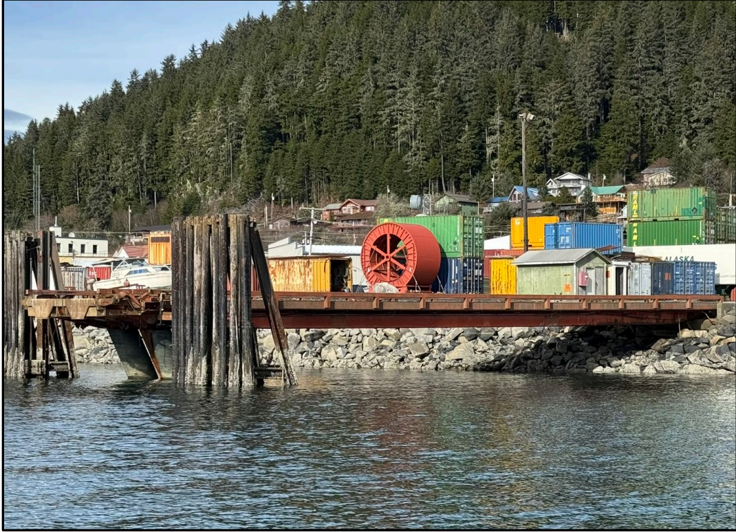
FIGURE 1. Overall view (south side looking north) of barge ramp.
