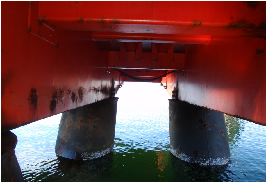
Ramp/support tank connection assembly.
