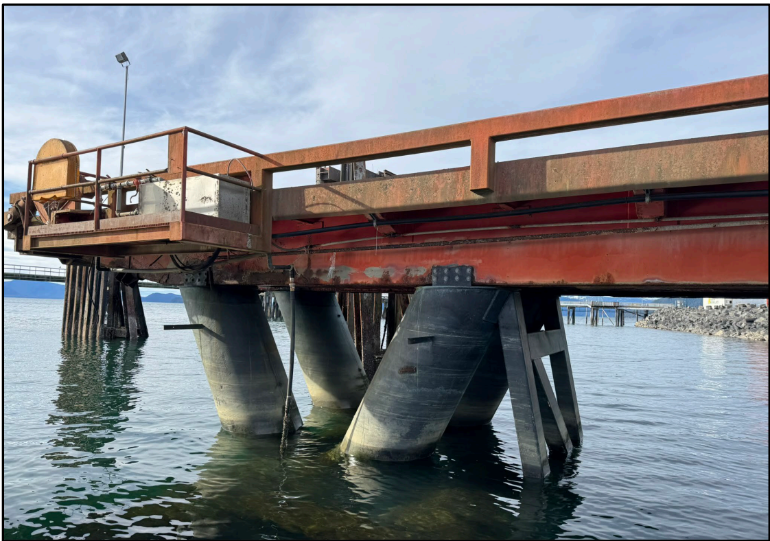
FIGURE 4. Floatation tank operation platform and ramp connection struts (south side).
