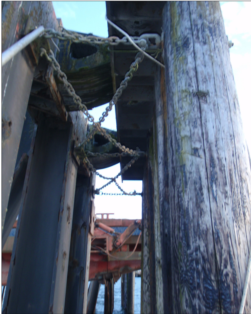
Original stay chain configuration at Dolphin "E".
