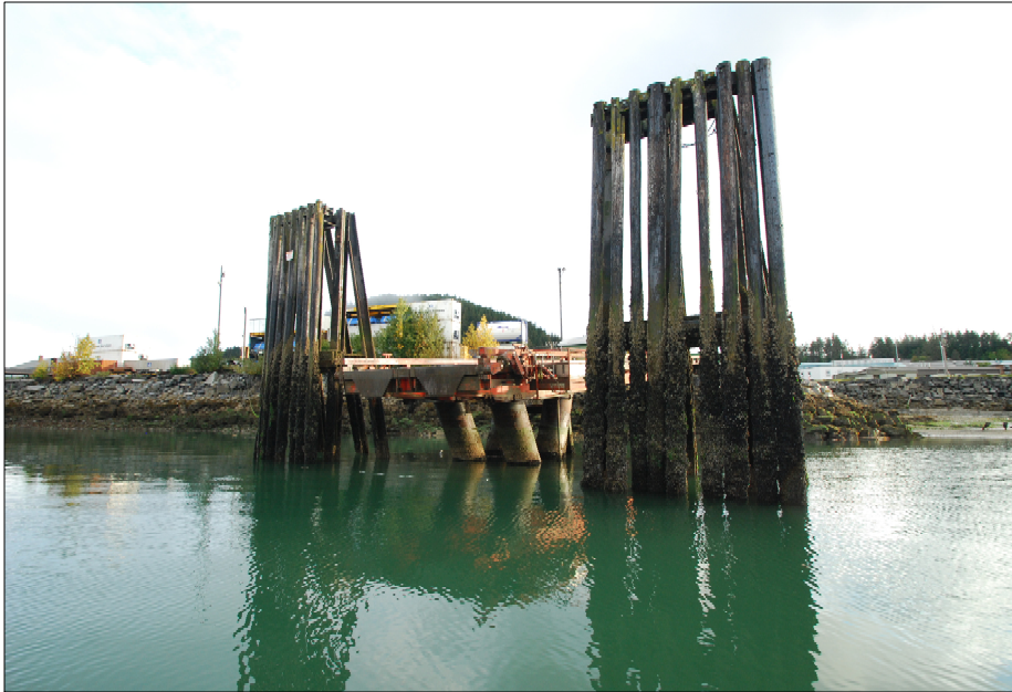
Barge ramp, looking north.
