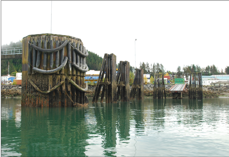
Overall view of barge ramp facility, looking east.
