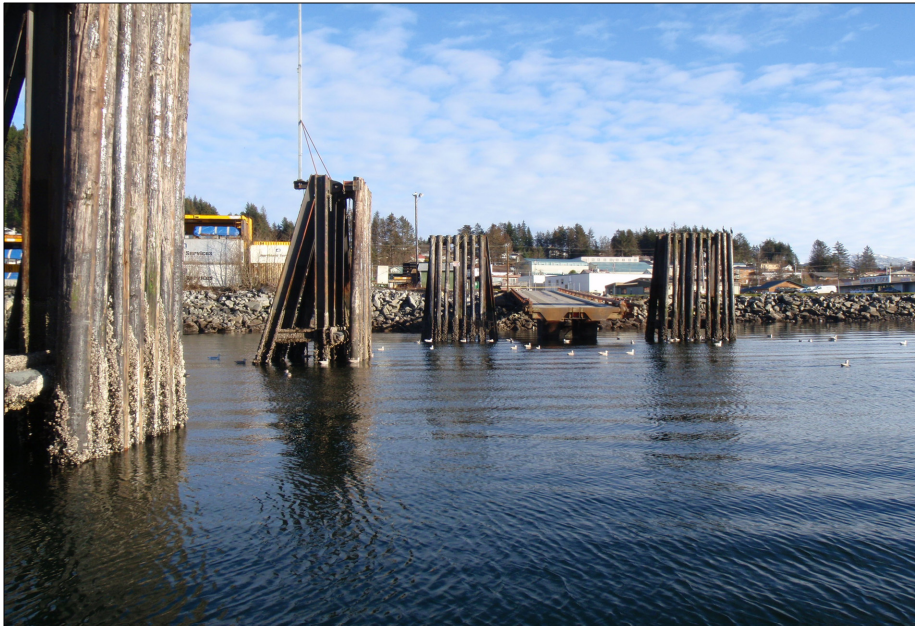
Barge ramp, looking east.
