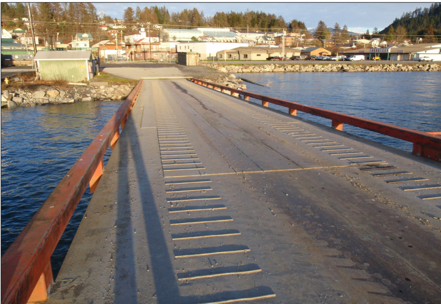
Top deck surface of barge ramp, looking shoreward.
