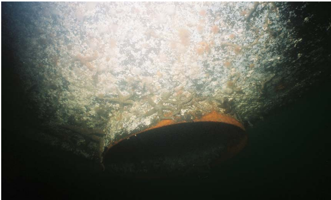
PHOTO No. 8: Floatation Tank Exhaust Port – Note the coating deterioration and minor surface corrosion on the bottom of one of the three exhaust ports located on the bottom of the 9 ft. diameter tank. Also note the good condition of the coating on the bottom of the tank.
