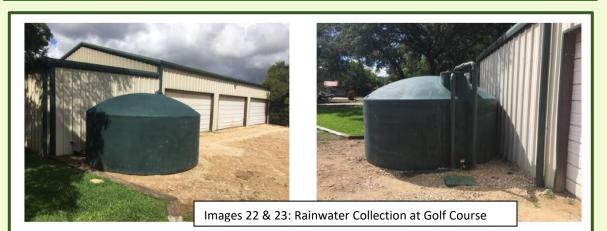
In 2018, the Cypress Creek Project team installed the above 5,000 gallon polyethylene cistern at the Woodcreek Golf Course. The cistern is collecting water off of a 2,700 square foot roof, which allows for the harvesting potential to be approximately 45,000 gallons annually. The rainwater harvested from this cistern is being used to clean golf carts at the facility.
