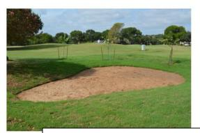
Work continued at the Woodcreek Golf Course in the summer of 2019, with the installation of this rain garden. Rain gardens are installed downslope of hills to capture stormwater. The bottoms are often planted with native plants to further treat the water before it recharges the aquifer.
