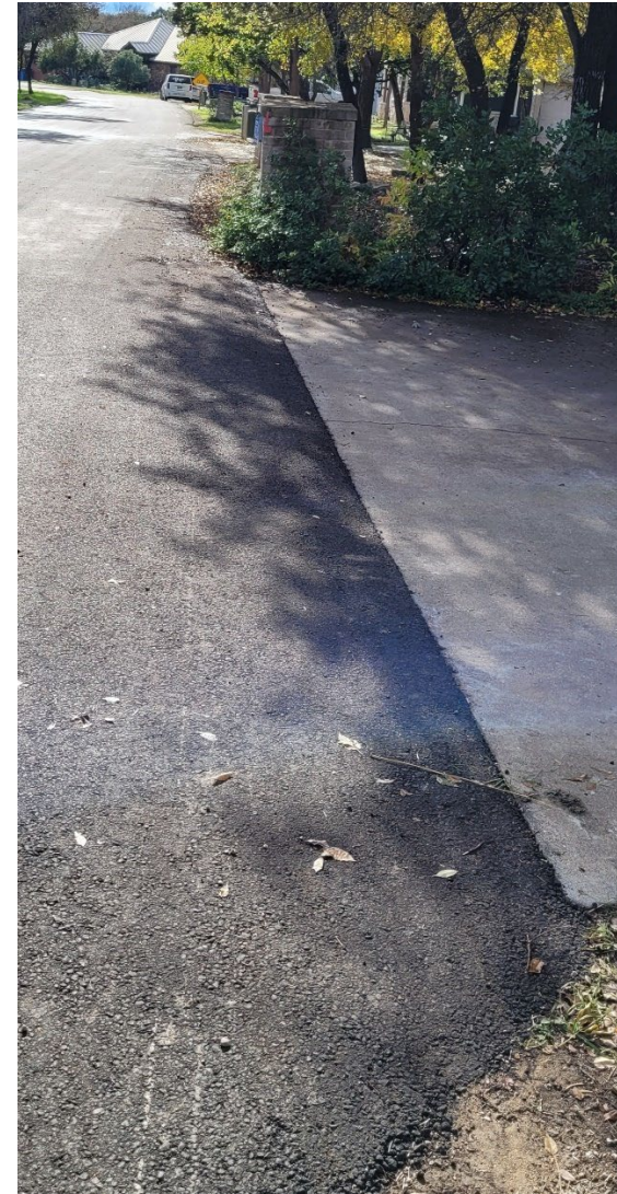
6 Canyon Creek / 8 Canyon Creek and 10 Canyon Creek - After
