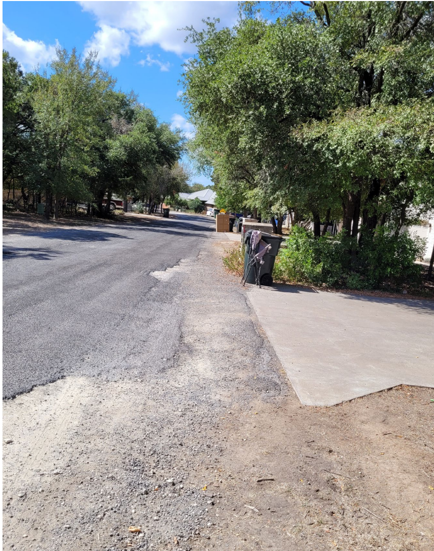
6 Canyon Creek / 8 Canyon Creek and 10 Canyon Creek - Before
