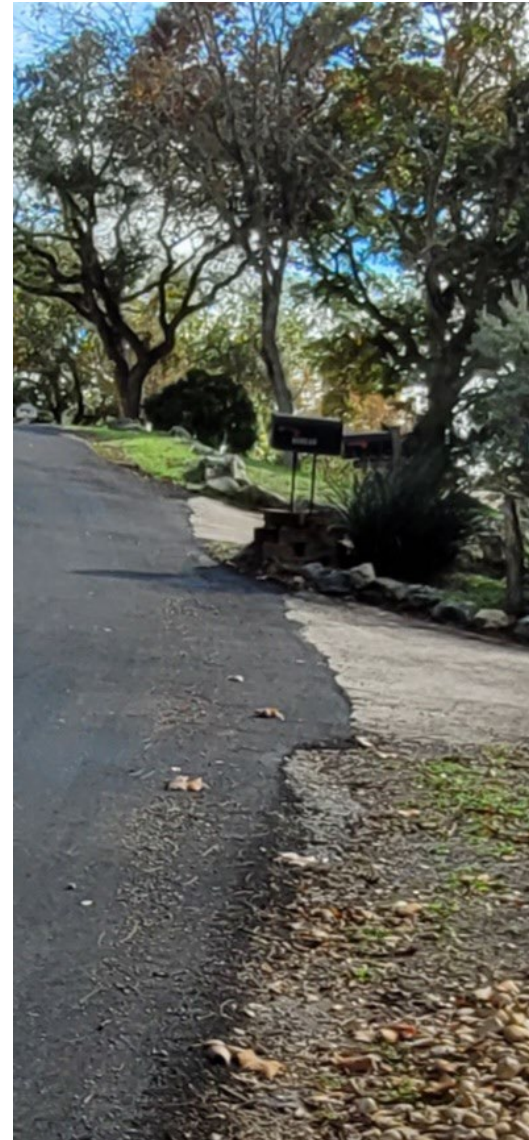
12 and 14 Tremont Trace - After
