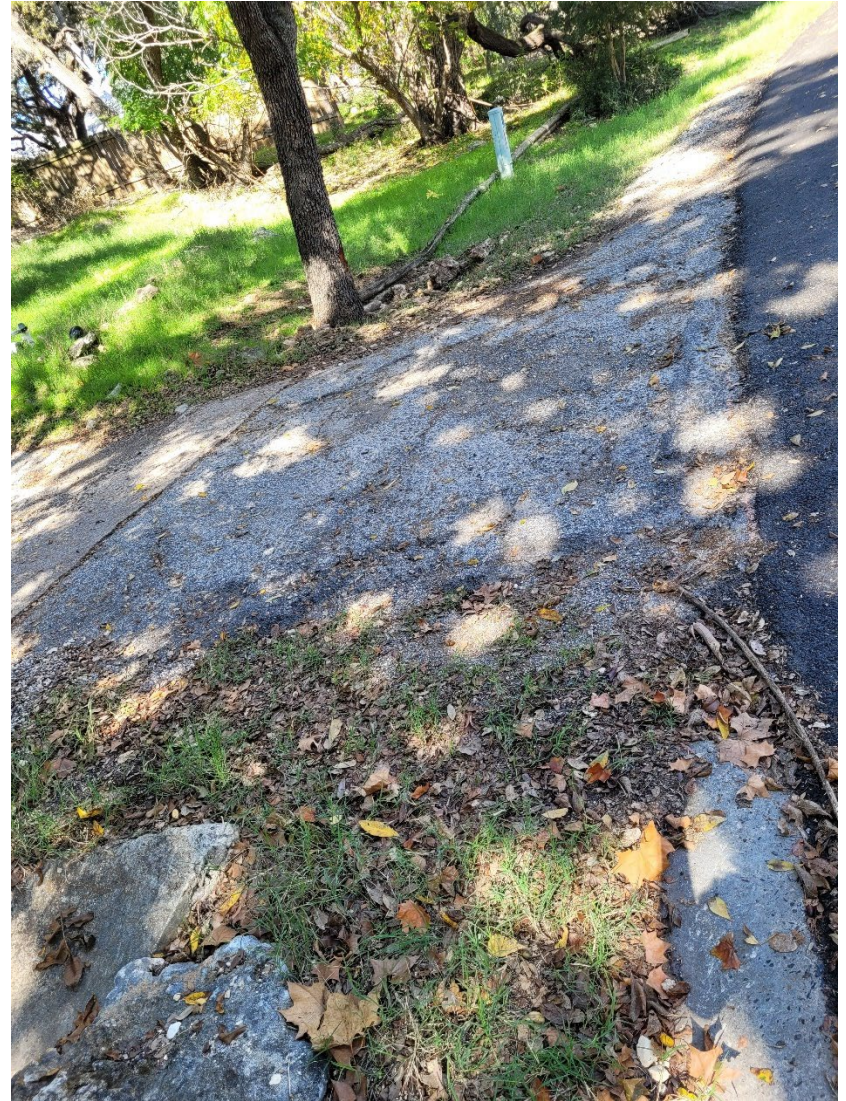
4 Tremont Trace – After (Asphalt Driveway & Approach)
