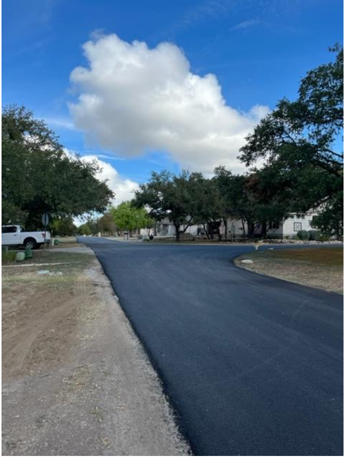
Doolittle Drive Facing NW
