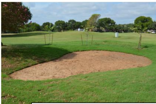
Image 24: Rain Garden on Golf Course at Installation
