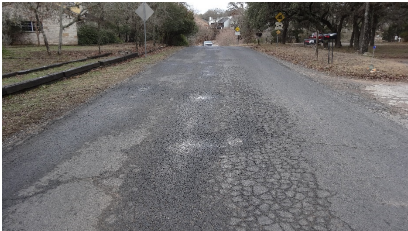
Figure 1: Alligator Cracks
