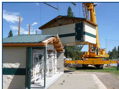
10 | Drop-In-Place Installation with a Crane
