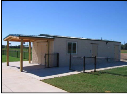
14' x 36' Restroom & Concession Facility
