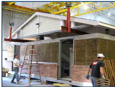
7 | Roof is Installed on CMU Walls
