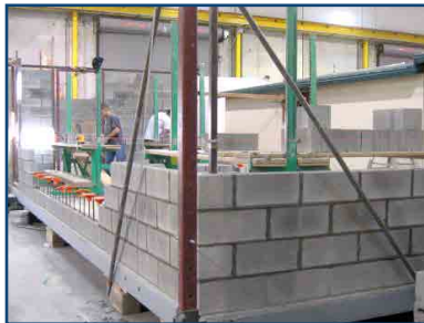
5 | CMU Walls Constructed on Concrete Slab
