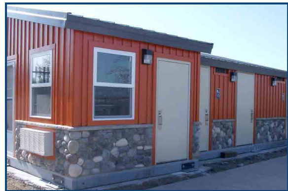
Laundry Room + Restrooms
