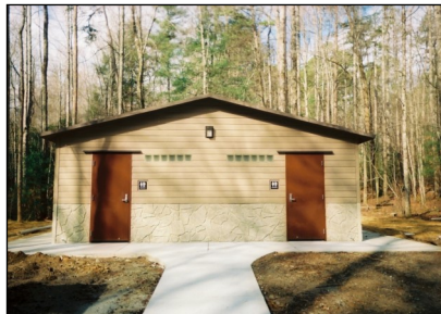
Men/Women ADA Restroom and Rear Showers
