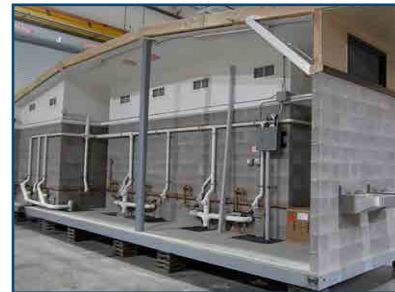
6 | Turnkey Electrical, Plumbing, and Fixtures
