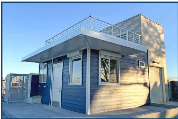
Lifeguard Station | Shower & Restrooms
