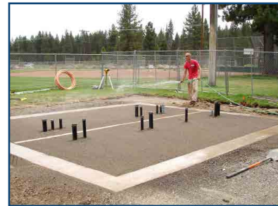
9 | Sub-Grade Pad Preparation
