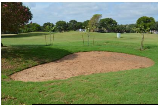
Image 24: Rain Garden on Golf Course at Installation
