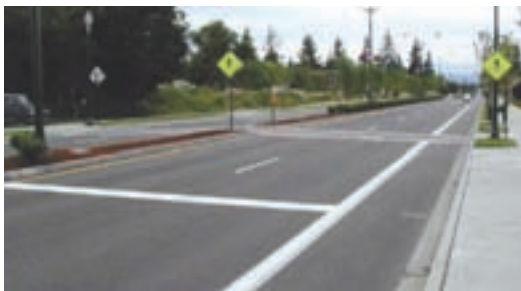
Advance stop lines can help prevent multiple threat pedestrian crashes.
