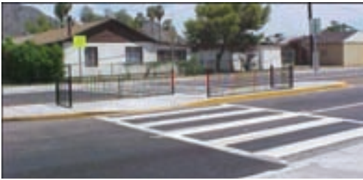
Two-stage crosswalks with fencing help direct pedestrians to look for vehicles coming from the right.
