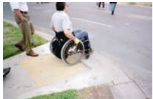
Well-designed curb ramps provide pedestrians with disabilities better access to the sidewalk system.
