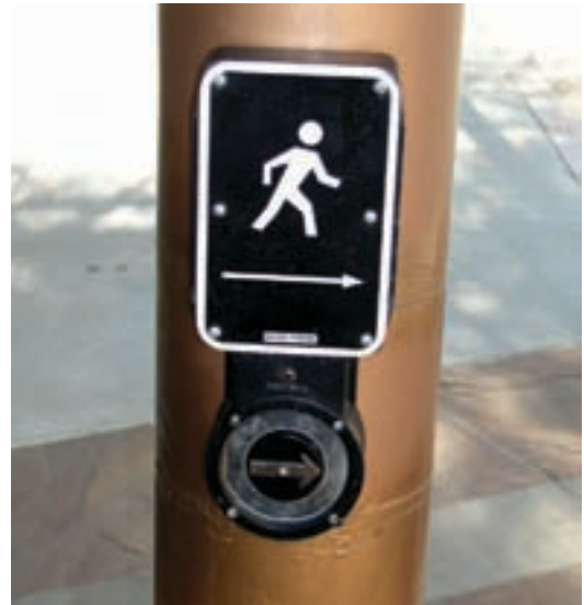
Push buttons such as this one should be placed where they can be easily accessed when waiting to cross an intersection.
