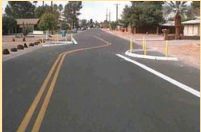
Traffic calming techniques, such as chicanes, were used in this targeted area to slow vehicle speeds on neighborhood streets.
