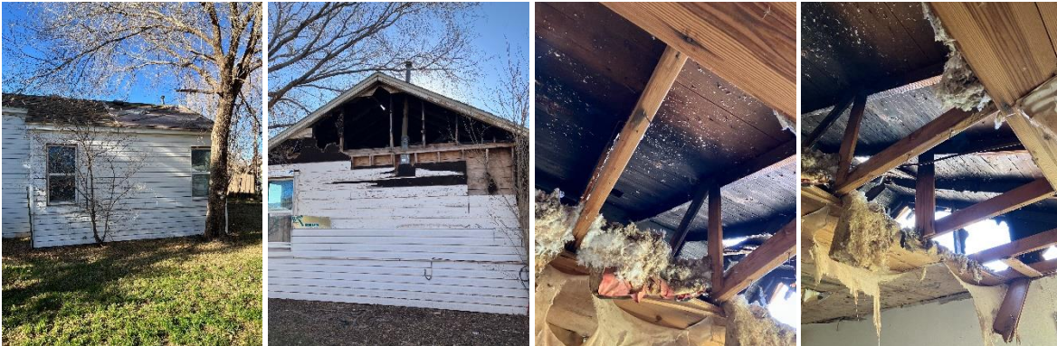
(19) Members of ceilings, roofs, ceiling and roof supports or other horizontal members, which sag, split, or buckle due to defective material or deterioration.
