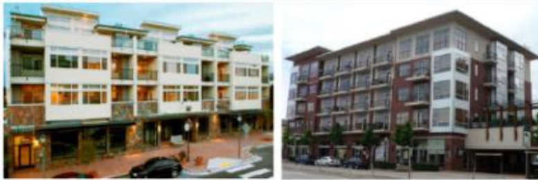
Images showing examples of appropriate building articulation
