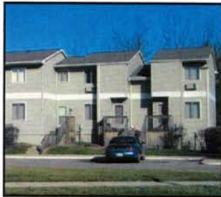
About 11% of Winnebago's housing stock is devoted to renter-occupied units such as the apartments shown above.
