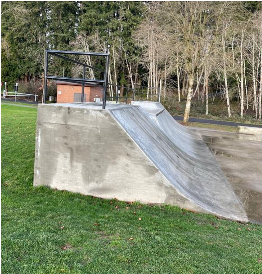
Wall 1 (side of wall 2)
