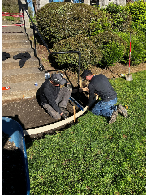
Forming Concrete Pad
