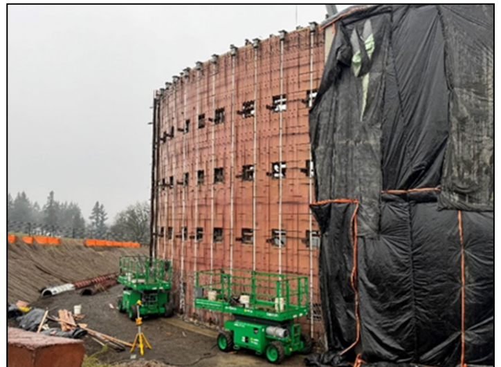
Reservoir wall forms prior to pour.
