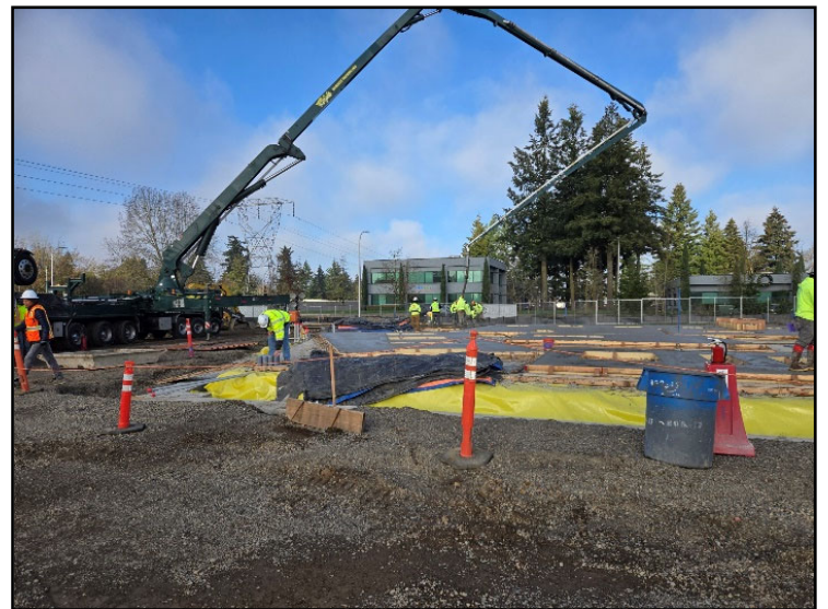
CIS office building site
