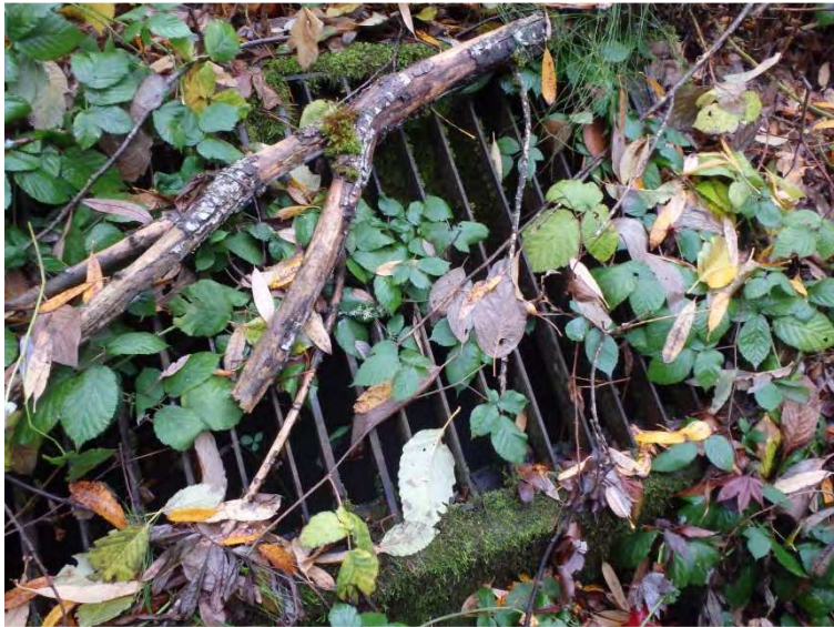
Photo 8 36-inch Outfall into Concrete Box
