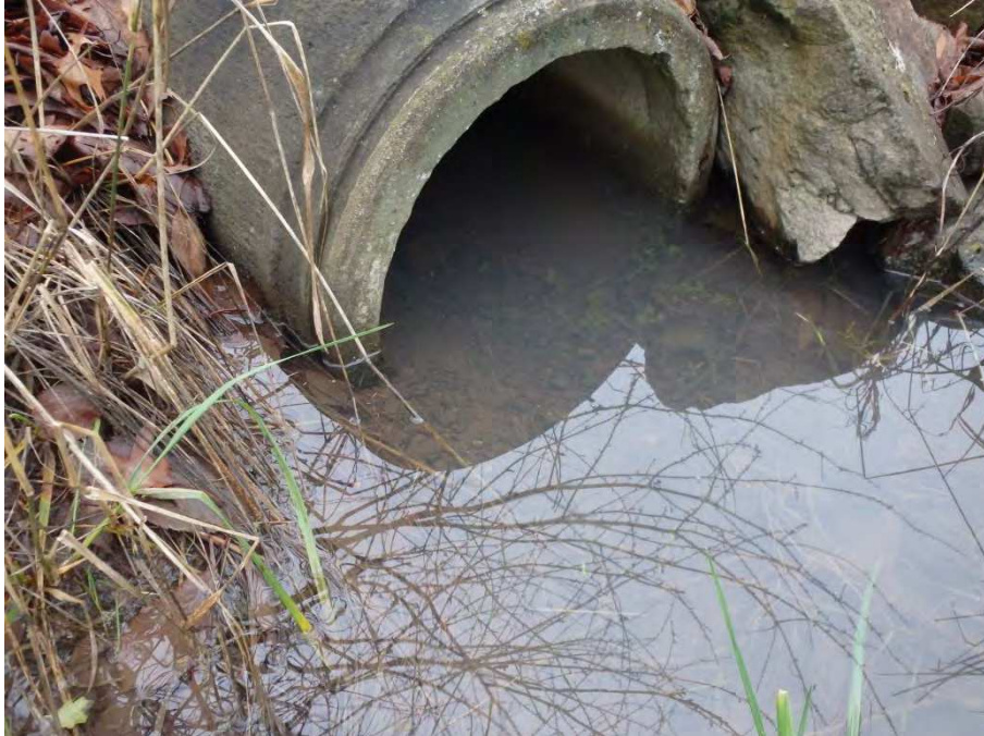
Photo 3 Downstream of culvert with gravel accumulation
