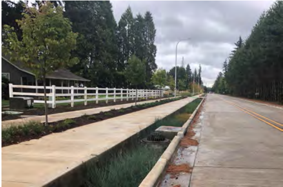
FIGURE 6: RECENTLY BUILT SIDEWALK AND CYCLE TRACK (EAST SIDE)
