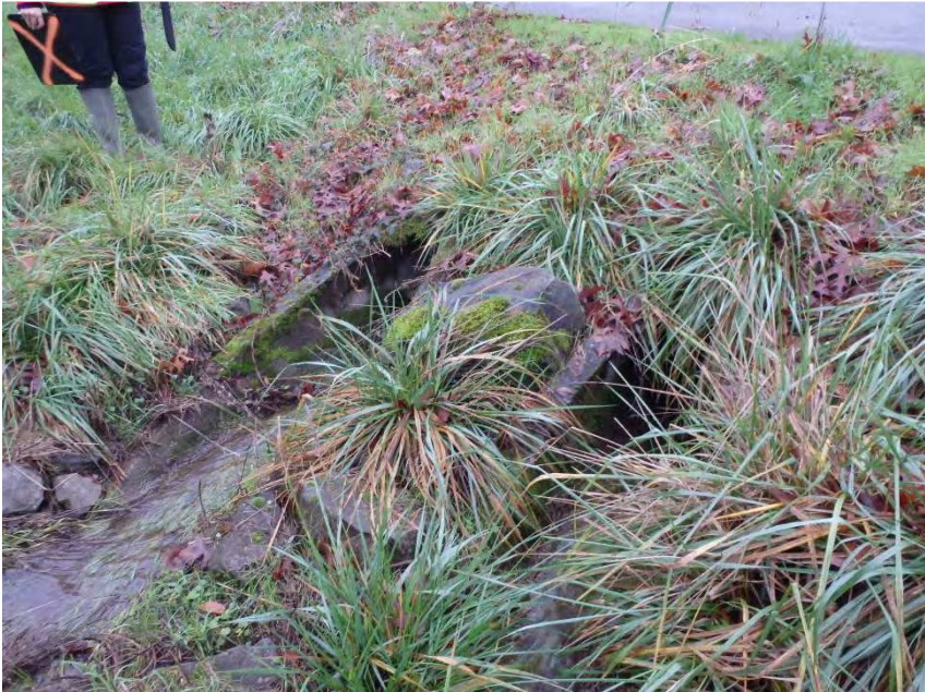
Photo 2 Upstream Ends of Culverts
