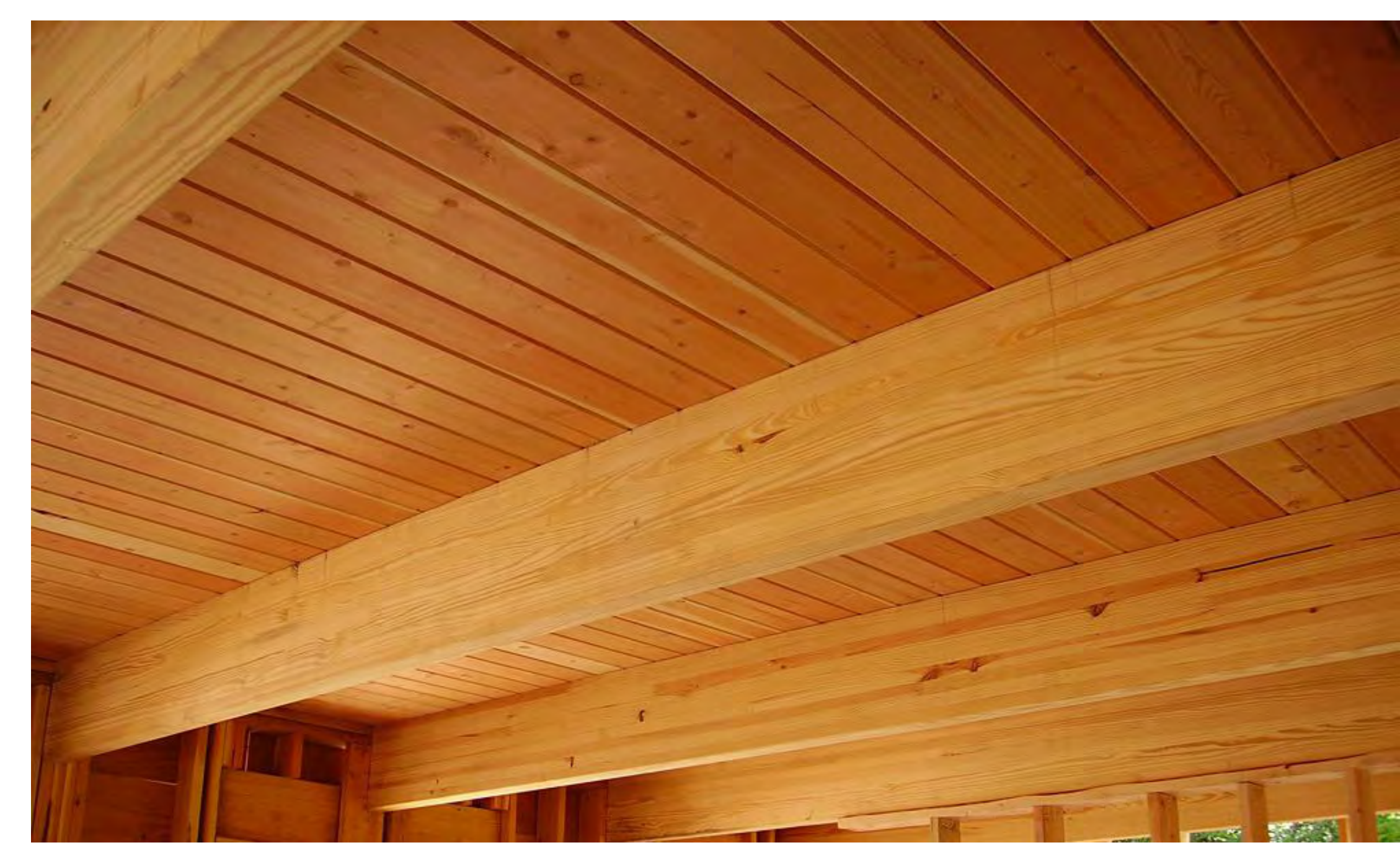
Canopy Structure and Decking
