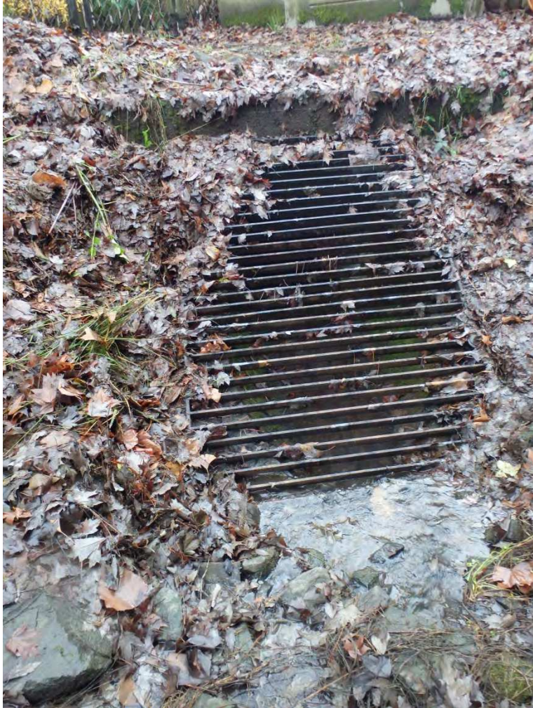
Photo 7 36-inch culvert under SW Willow Creek Drive
