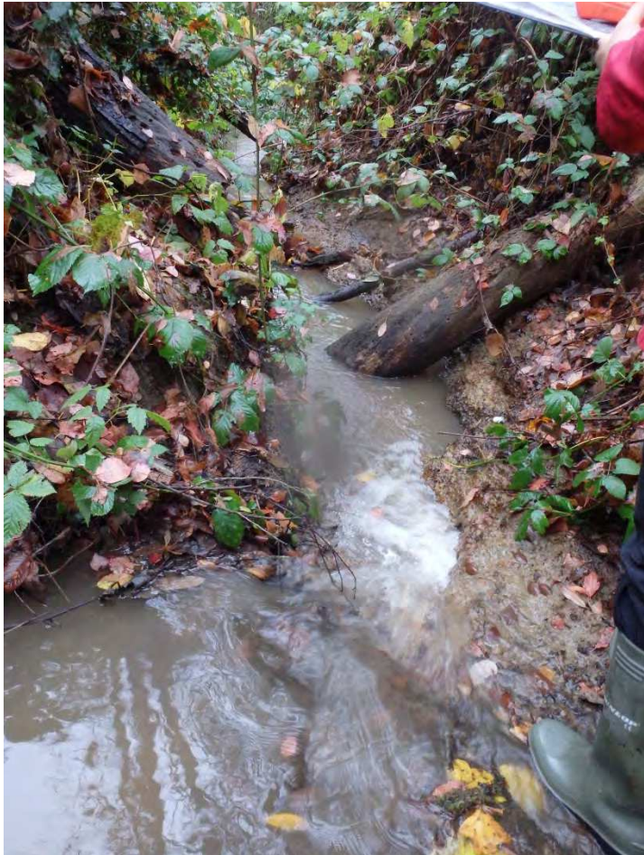
Photo 15 2-ft high drops in Channel
