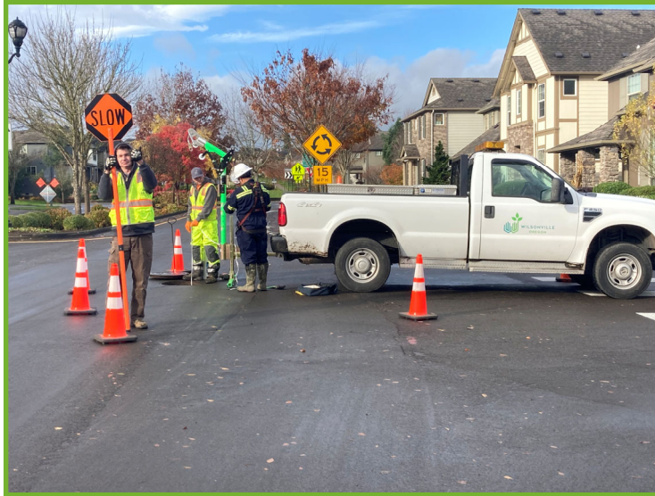
Paul flagging during a manhole repair
