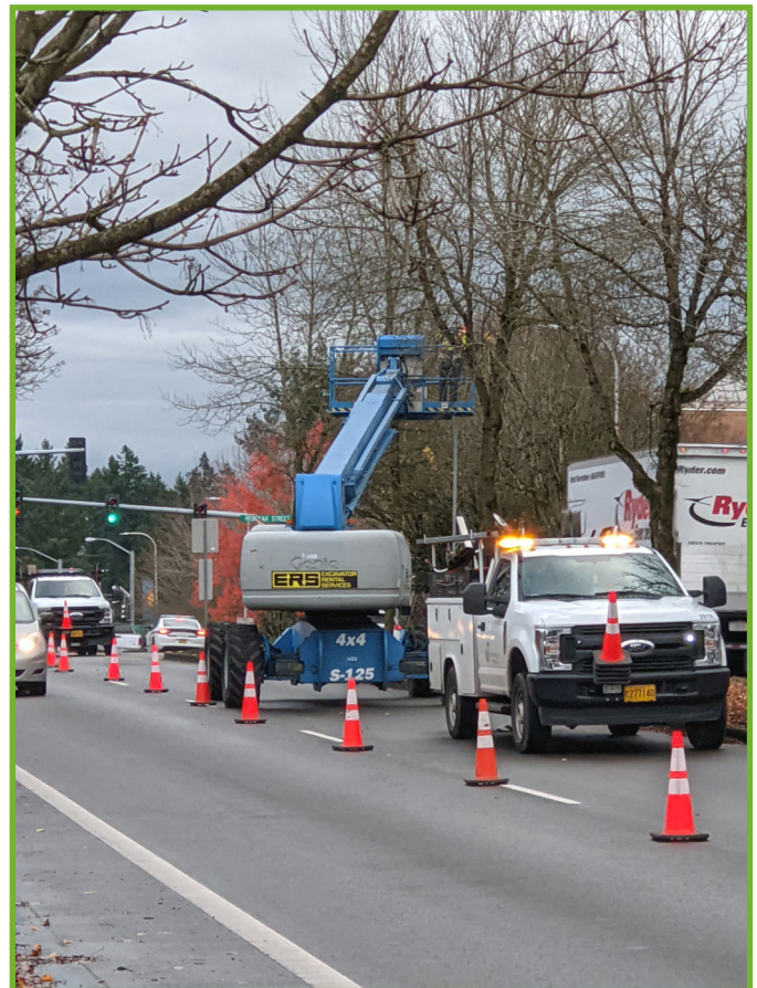
Working safely in the roadway
