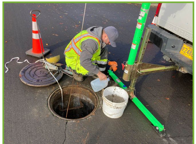
Randy mixing patching material
