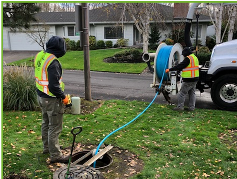
Jetting the line to remove debris
