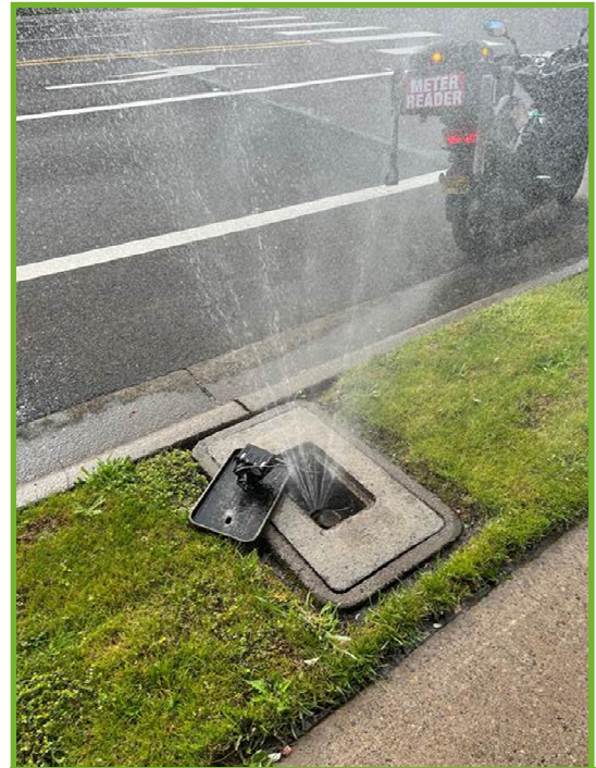
Leaky meter on Main Street
