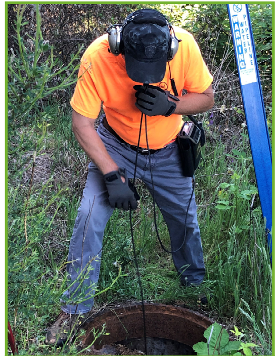
Leak detection in progress
