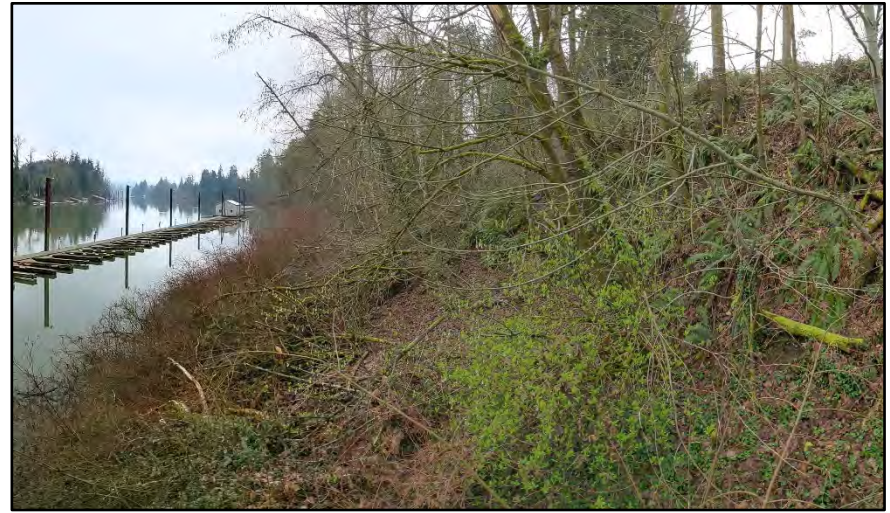
Photograph B-6. Photograph looking east along the Willamette River. Photograph taken 3/7/2022.
