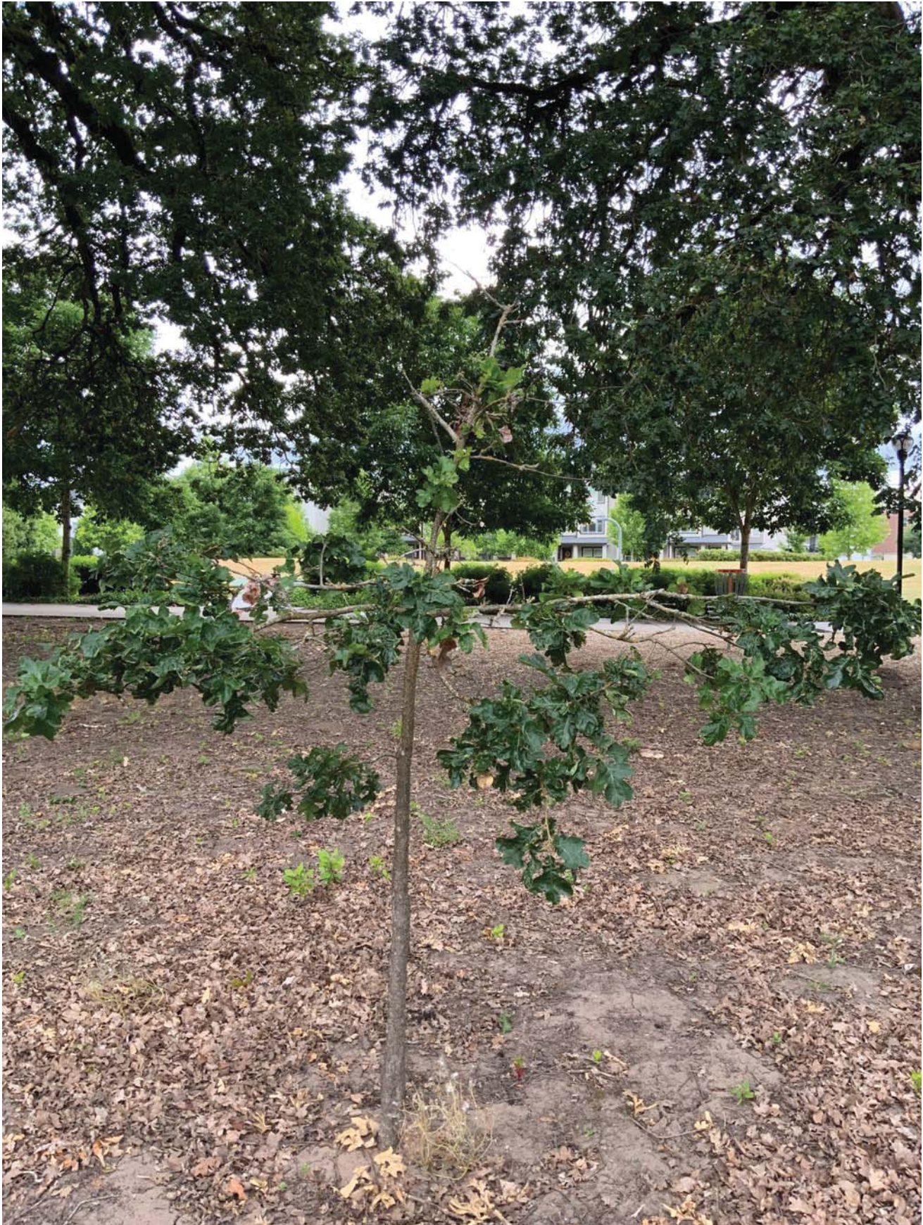
Photo 7. Tree #25818 - Small oak with dead top, lower trunk damage, wilted leaves, small live crown could be replaced sooner than later.
