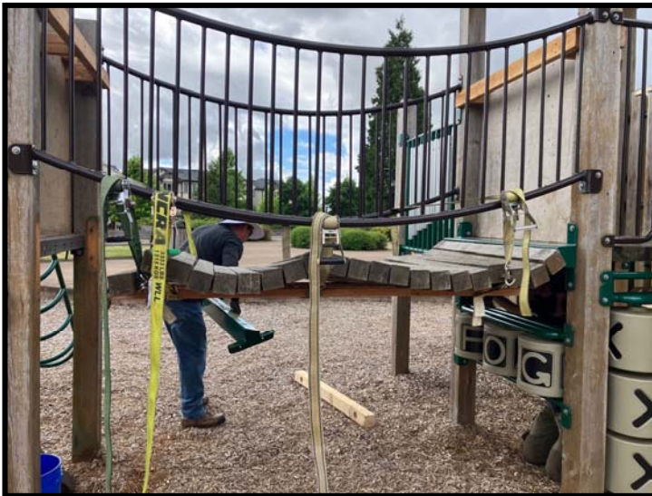
Team making playground repairs at Edelweiss
