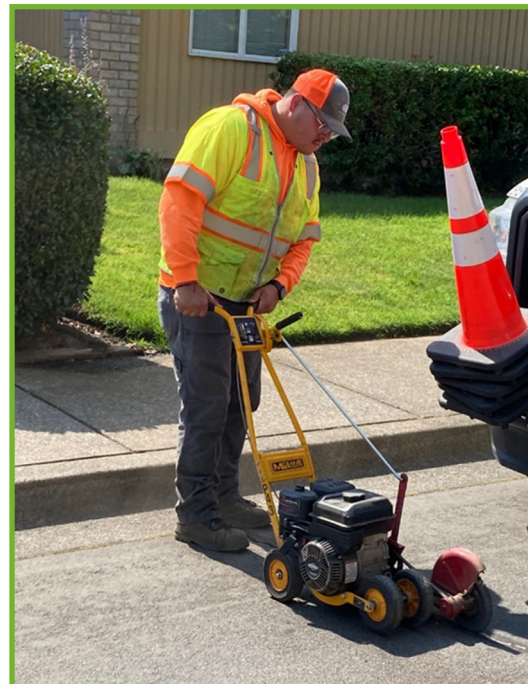
Eric doing prep for slurry seal
